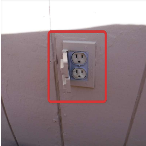
No GFCI at exterior back of house on deck. No GFCI at front exterior of house.
