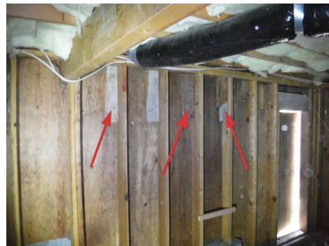
Blocks across the back where hanger nails from deck joists.
