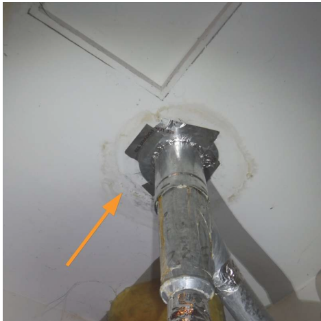
Same vent in garage with ring of
