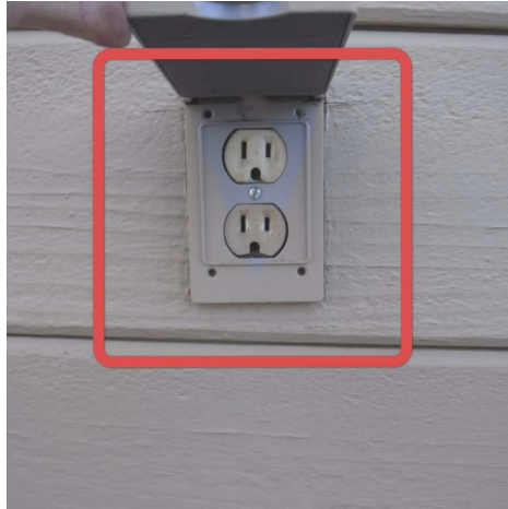
No GFCI at exterior back of house on deck. No GFCI at front exterior of house.
