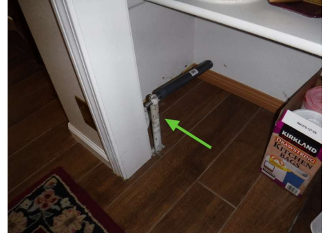
Water shut off. Inside closet by garage entry to house.
