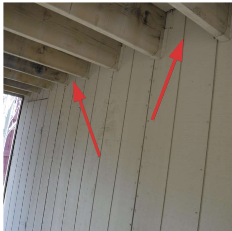
Blocks across the back where hanger nails from deck joists.
