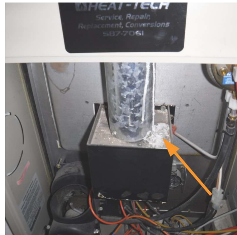
Water entering from gap in roof vent.
