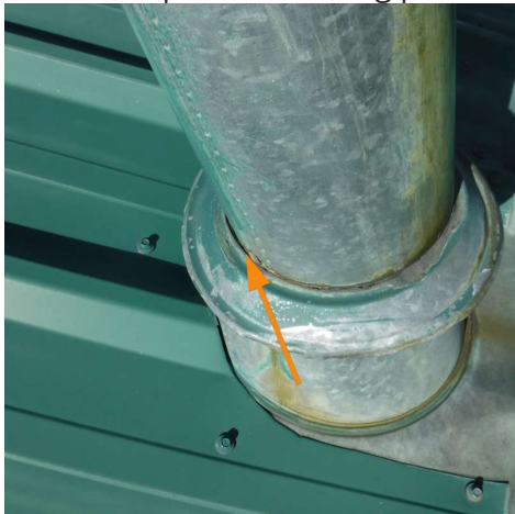
Gap in waterproofing
