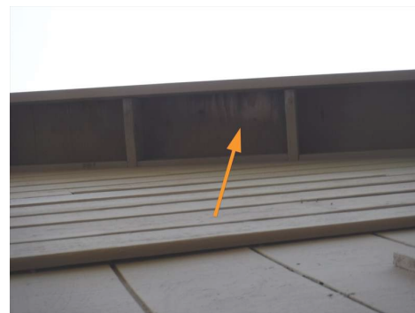
Eave on left side of house
