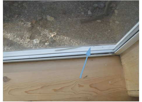
Outside of picture window in dining area.
