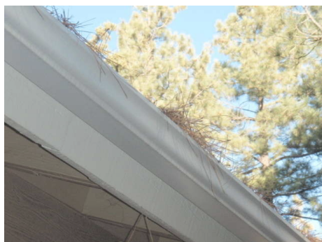
Gutters containing debris
