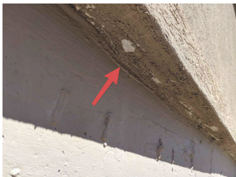
No clear drainage plane
