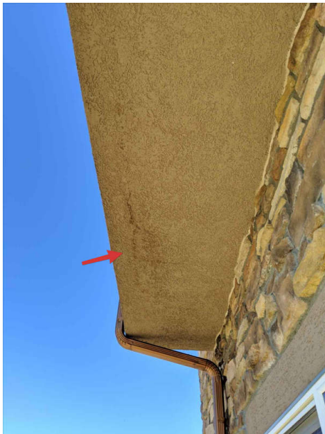
Moisture staining under west window
