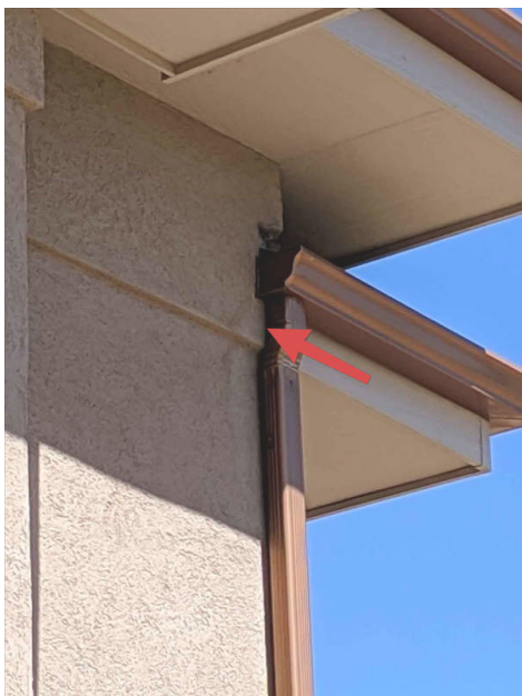
No clear drainage plane
