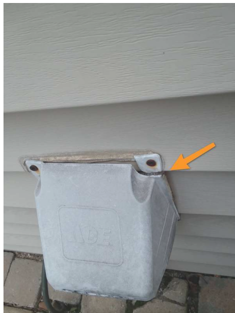
Cracked at top
