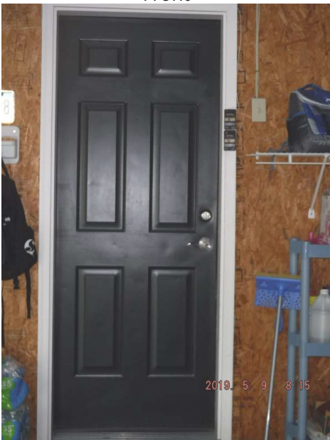
Garage to Pool Area
