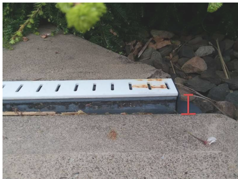
Approx. 1-1/4" difference in height between slabs.
