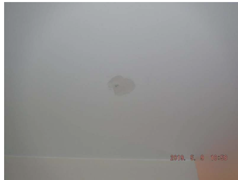
Ceiling Repair Needed
