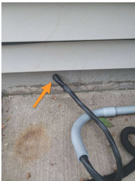
Wire taped but no adequate weather or human protection.
