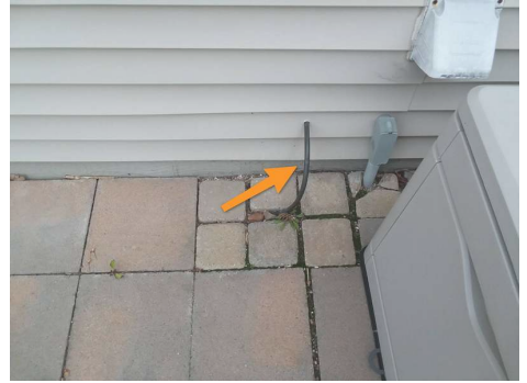
Copper pipe enters house
