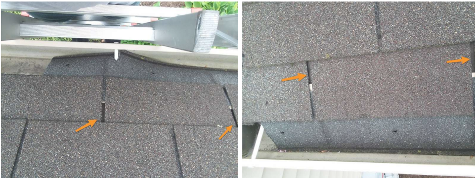
Underlayment exposed at water ways
