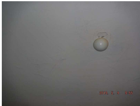
Wall Repair Needed
