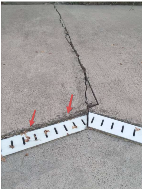
Approx. 3/4" height difference between slabs
