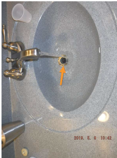
Drain stopper missing
