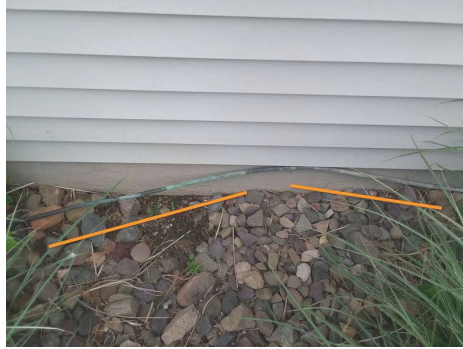
Copper pipe continues along planting area
