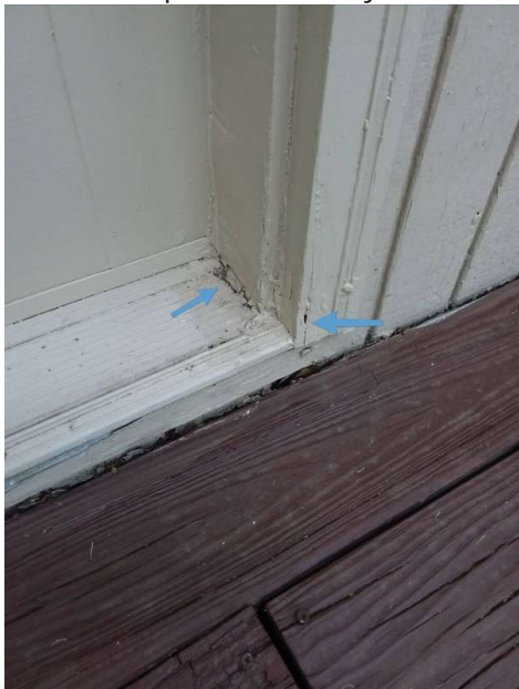
Exterior door at top deck
