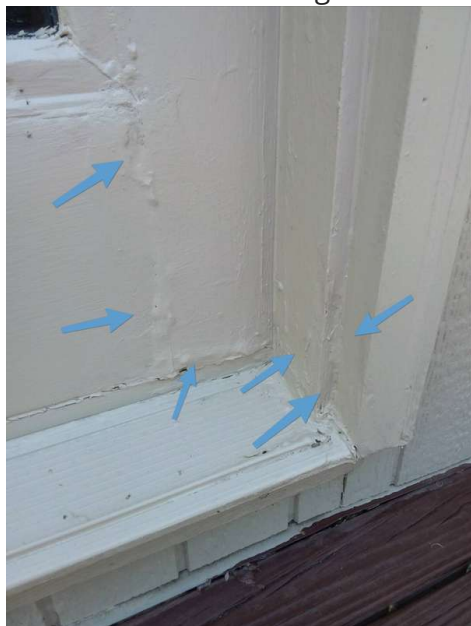
At main deck
