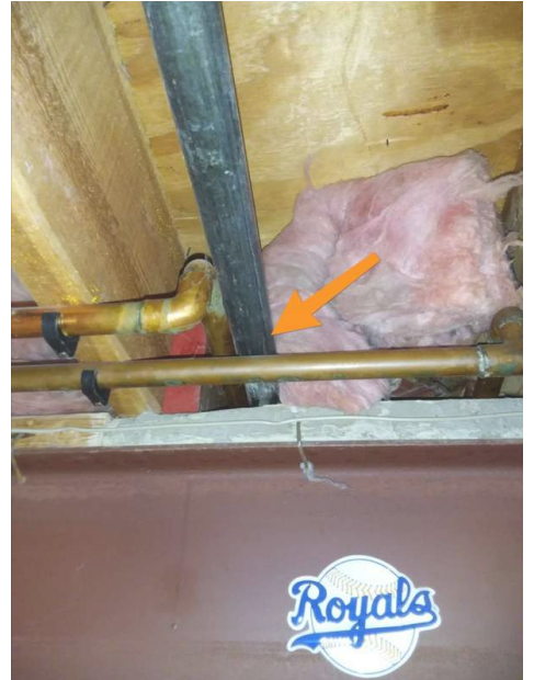
Above furnace room Basement
