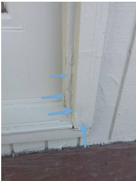
At main deck
