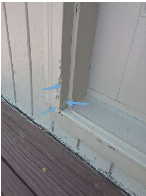
At main deck
