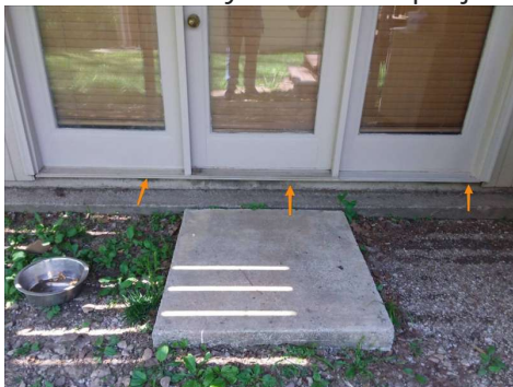
Lower level back door
