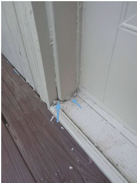
Exterior door at top deck
