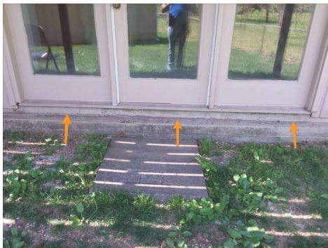
Lower level back door
