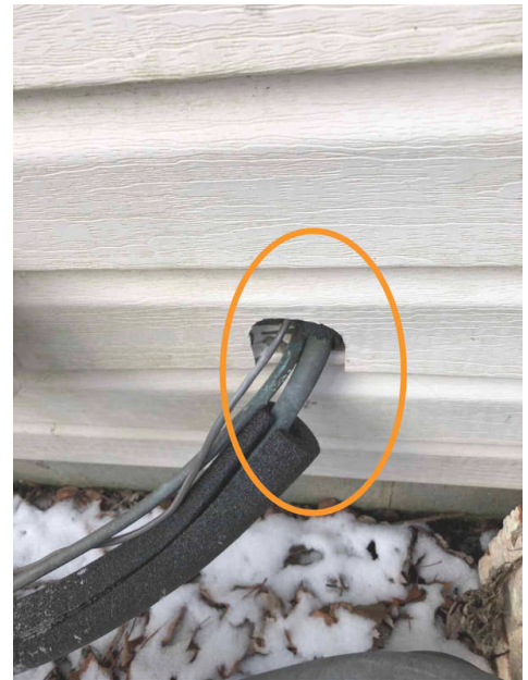
Missing insulation
