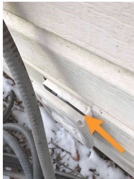
Dryer vent- East
