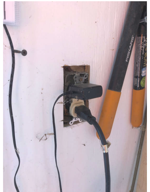
Garage-east of overhead door
