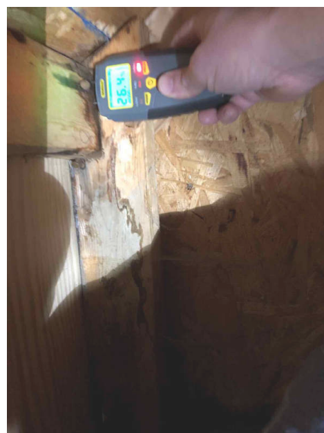
East Garage Attic-near access
