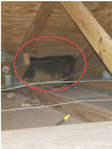
Evidence of previous roof leak as seen from the attic.
