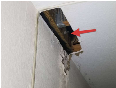
Previous repair from leaking roof. Recommend roofing professional for further evaluation.
