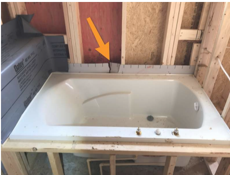
Damaged "Draft-Stop" Rigid Board
