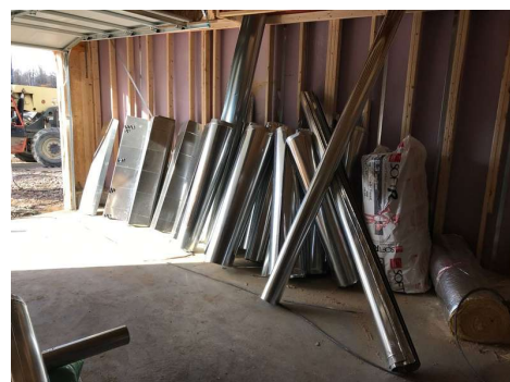
Slab Partially Blocked By Building Materials
