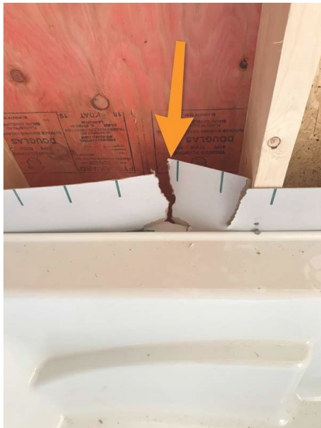
Damaged Draft Stop Board
