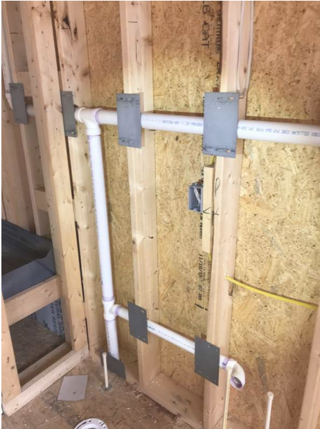
Nail Guards Installed
