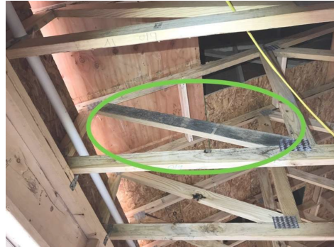
Suspected Mold Above 3rd Floor Bedroom (Front)
