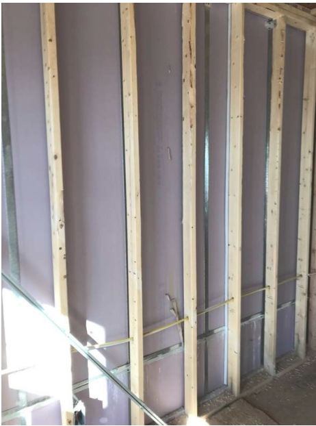
2 Hour Rated Fireblock Installed
