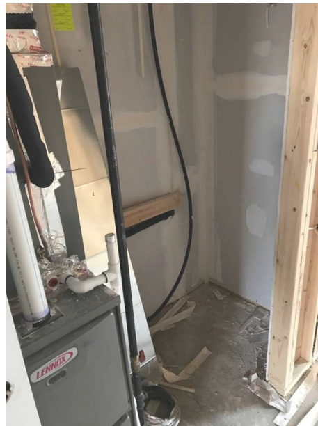
Location For Gas Water Heater (No Water Heater Present)
