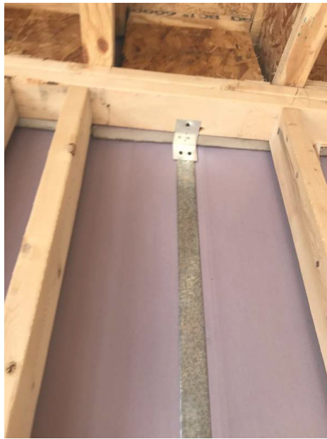
Fireblocks and Fire Stops Installed
