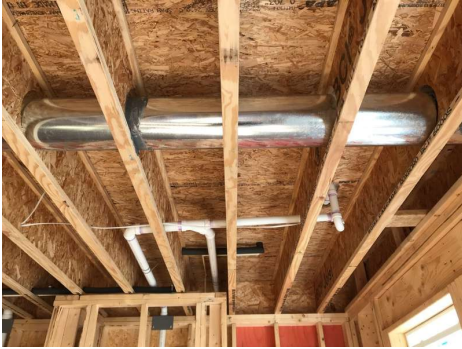
Engineered Truss Flooring / Ceiling
