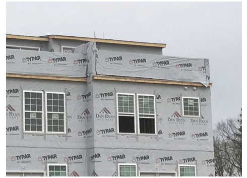
Gutters Not Installed
