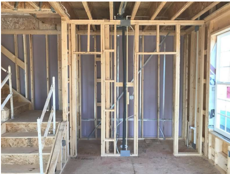
Walls / Dimensional Lumber Plumb
