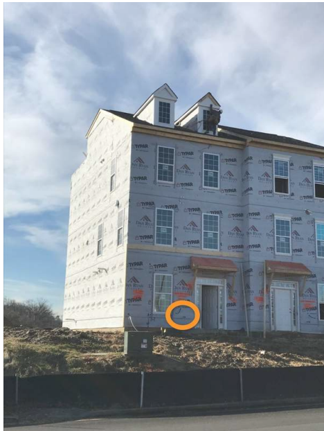
Front Hose Bib Loose
