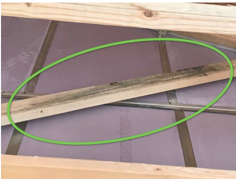
Suspected Mold Above 3rd Floor Bedroom (Front)
