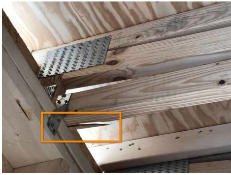
Damaged Chord Truss
