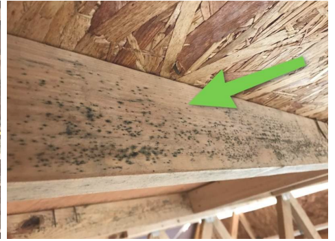
Suspected Mold On Roof Truss
