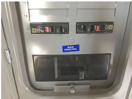
Circuit Breakers Partially Installed
