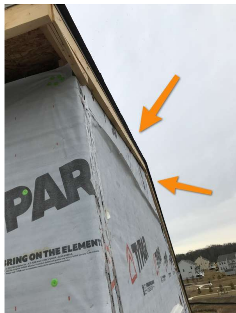
Missing House Wrap Tape
