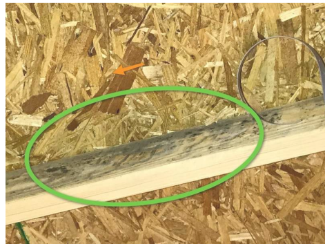
Suspected Mold On First Floor Truss
