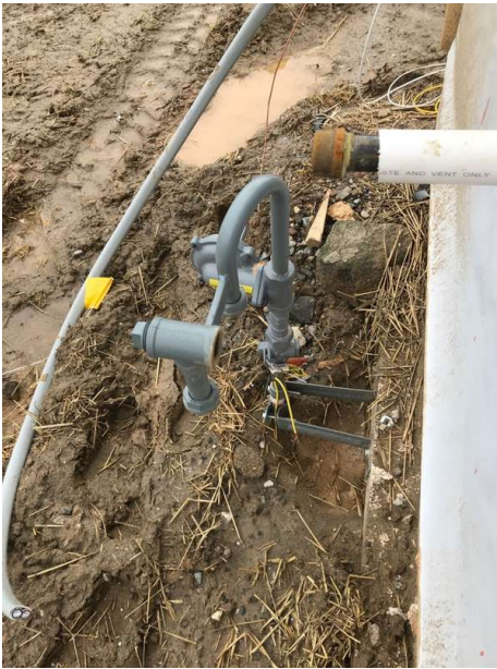
Location For Gas Meter (Not Installed)
