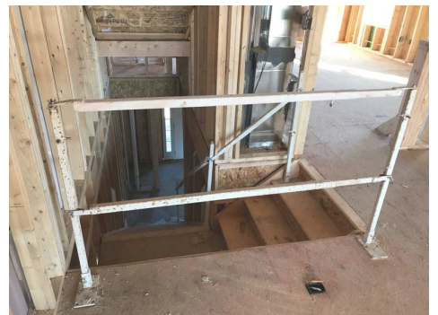
Temporary Railings In Place
