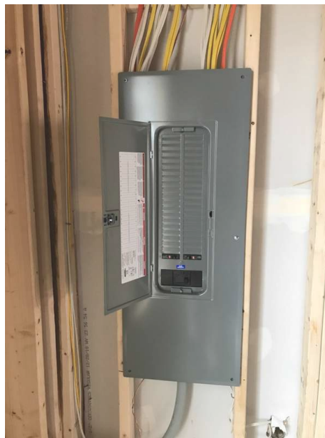
Main Electrical Service Panel
