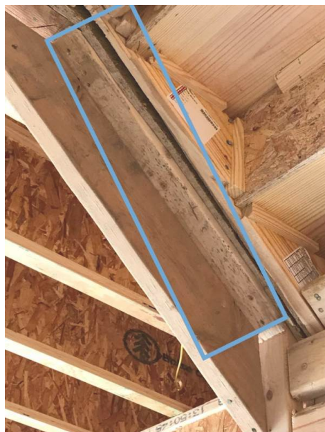
Bio-Growth In Garage Adjacent To Stairs
