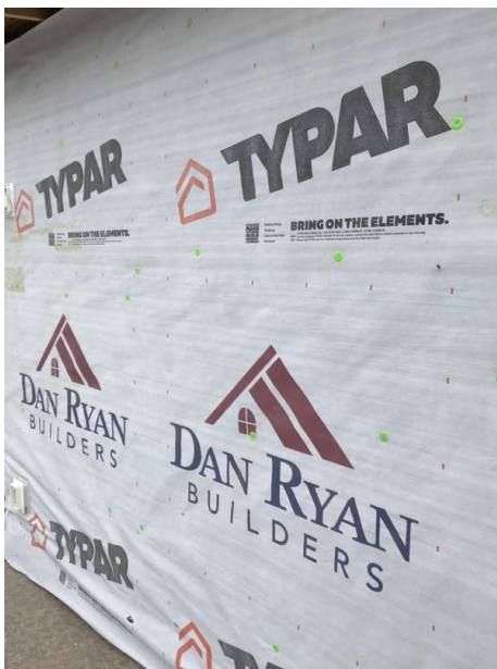
OSB Sheathing With Typar House Wrap
