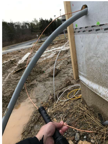
Copper Ground Wire Present, Not Yet Connected To Grounding Rod
