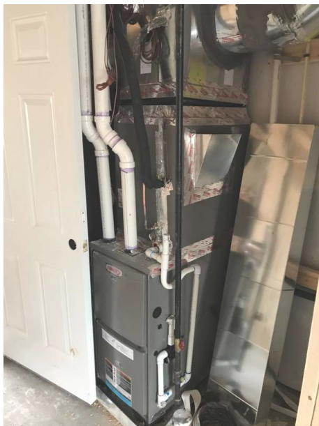
High Efficiency Gas Furnace
