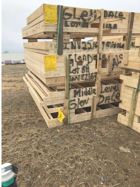
Trusses Stored With Ground Contact / Uncovered
