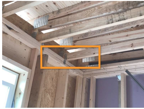
Damaged Chord Truss In Master Bedroom
