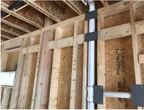
Kitchen Cabinet Blocking
