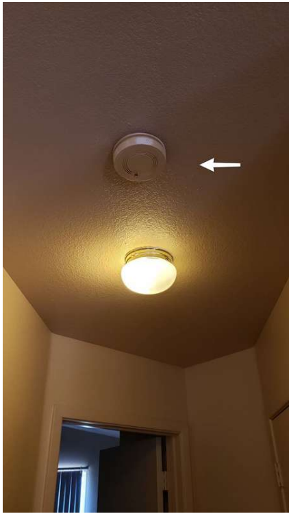
Hallway - 2nd Floor
