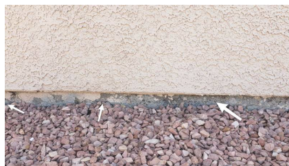
Garage - Right Side
