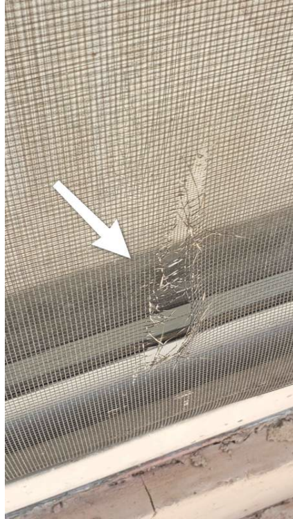
Sliding Door to Patio
