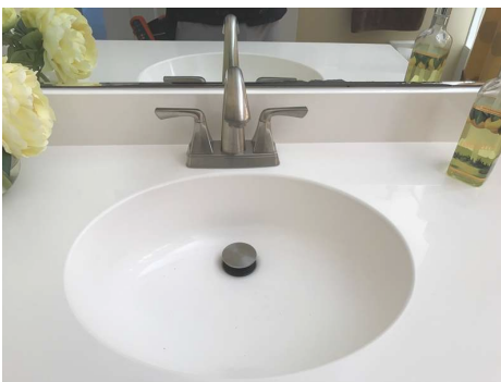
Sink/countertop: Sink Plumbing Photos
