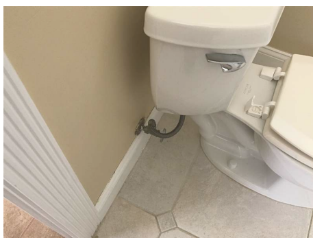
Toilets: Toilet Plumbing Photo
