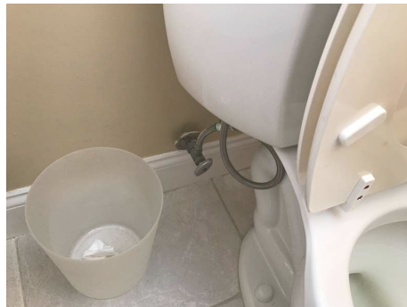
Toilets: Toilet Plumbing Photo
