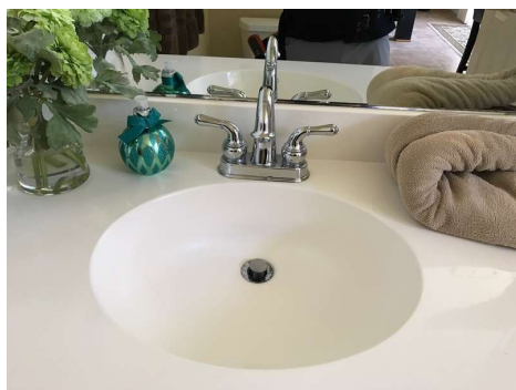
Sink/countertop: Sink Plumbing Photos
