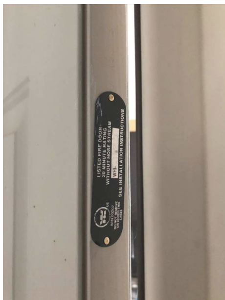
Garage entry door. Fire rated 20-minutes.
