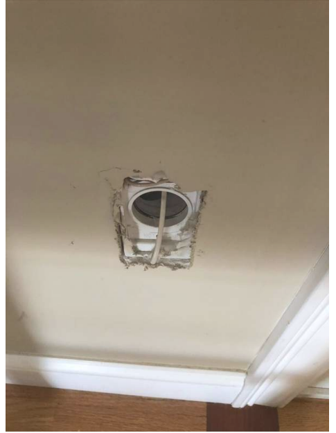
Main floor entry way. Missing cover plate.
