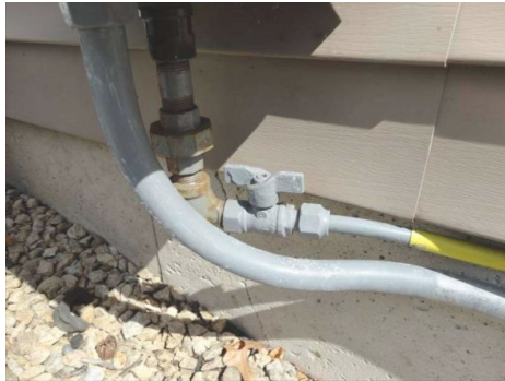
Exterior gas shut-off valve located on west side of home.
