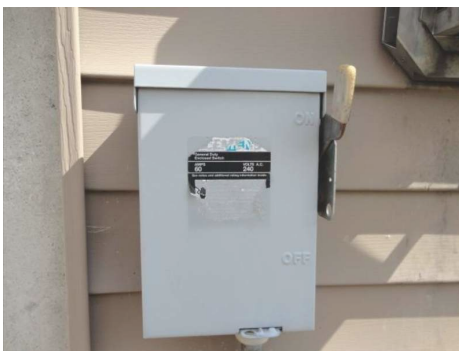
A/C main shut-off
