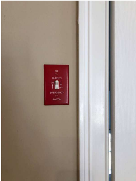
Oil Burner emergency shut-off switch located in kitchen against south wall.
