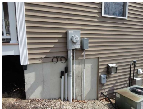
Underground service lateralSouthwest
