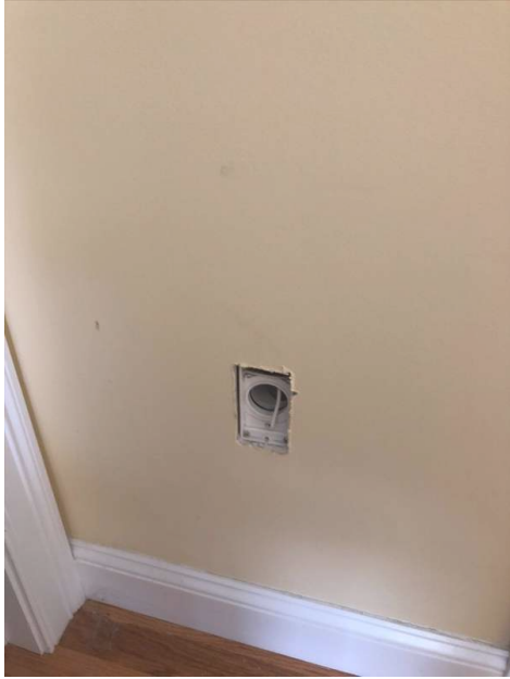
2nd Floor hallway missing cover plate.
