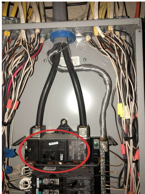
Main disconnect. Located in basement utility room. Basement
