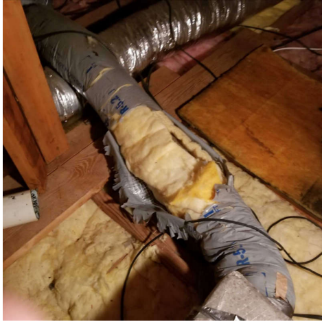
2nd Floor Attic
