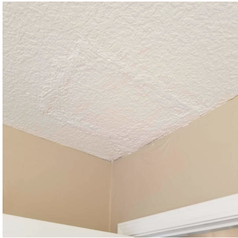
1st Floor Bedroom
