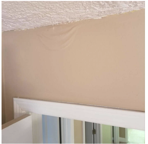
1st Floor Bedroom
