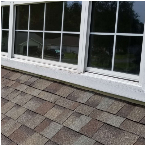
Front window 2nd Floor
