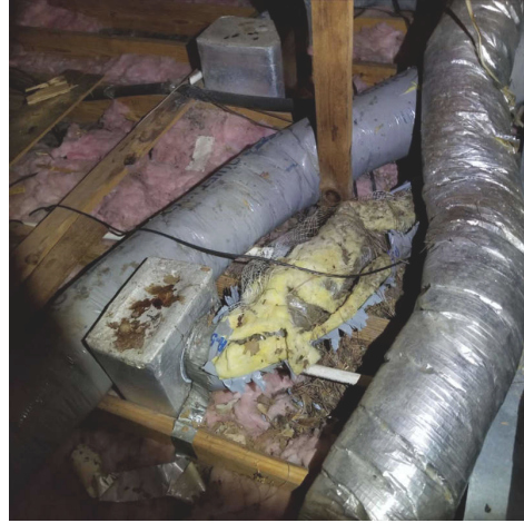
2nd Floor Attic
