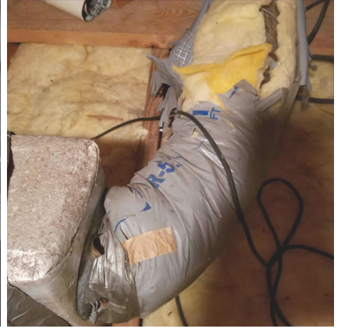
2nd Floor Attic
