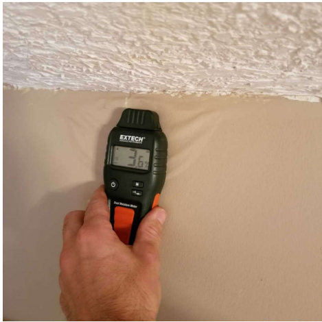
1st Floor Bedroom
