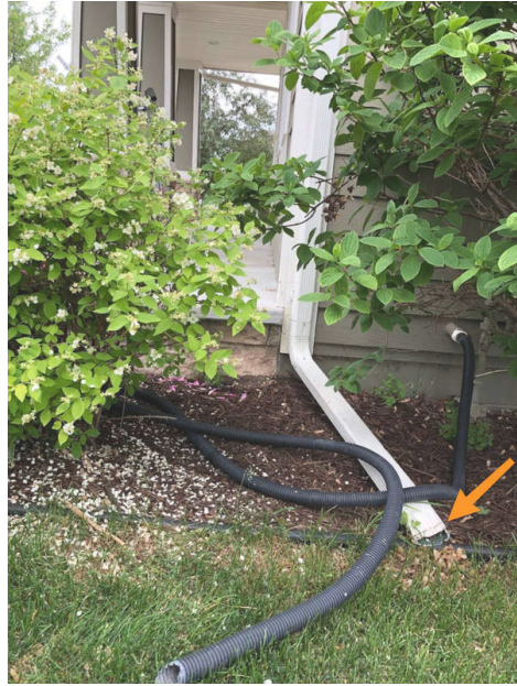
Repair - Recommend that extensions carry water out 4-6 feet from the house. Repair and extend
