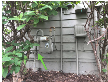
Outside Shut Off
