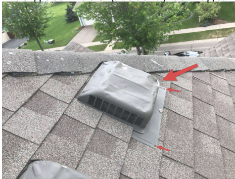
Damaged Vent and no Calk to seal the nail heads.
