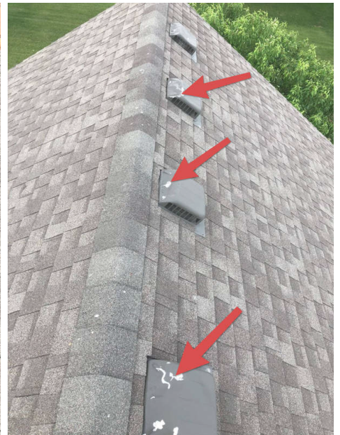
Damage on the vents.
