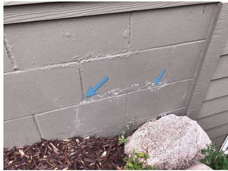
Minor cracking with efflorescence.
