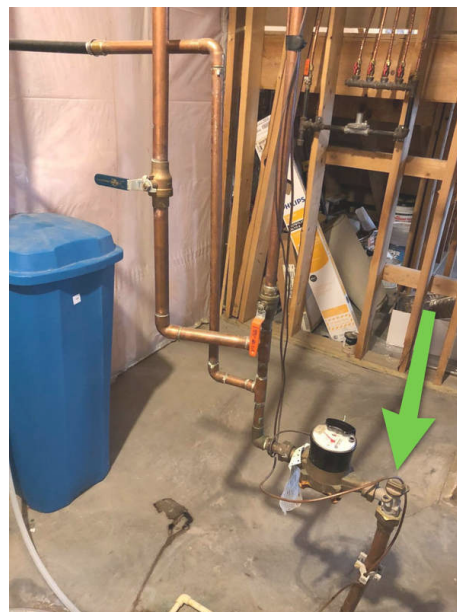
Main ater shut Off
