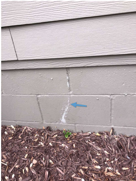
Minor cracking with efflorescence.
