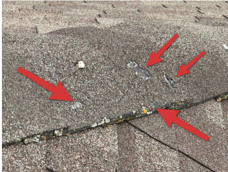
Fiberglass mat exposed by damage.
