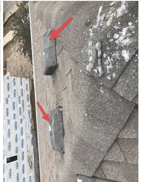
Damaged Vent and no Calk to seal the nail heads.
