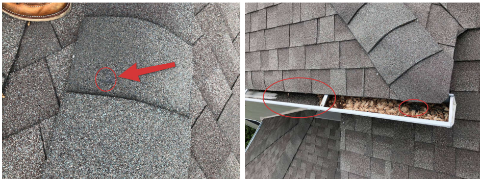
Significant aggregate washed off the shingles.
