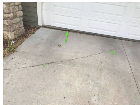
Minor cracking and settling.
