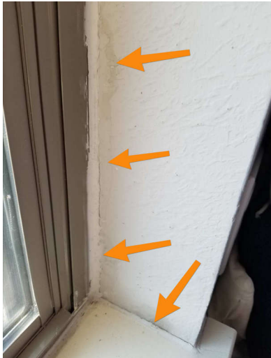
2nd Floor Northeast Bedroom
