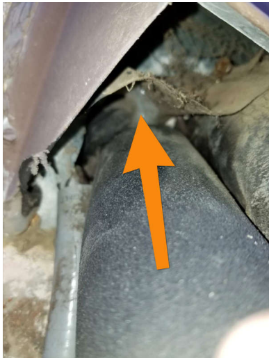
AC Lines South Exterior
