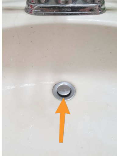
2nd Floor Bathroom
