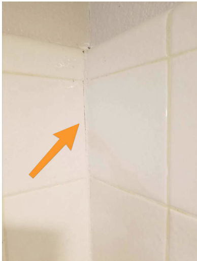
2nd Floor North Bathroom
