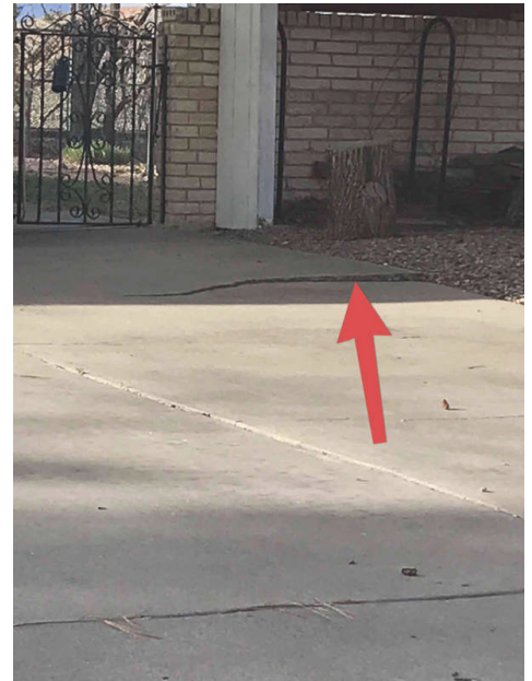
The large tree is causing this.
