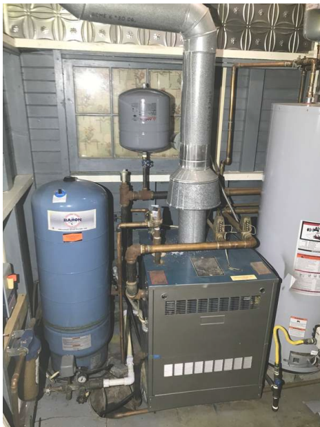
Burnham Steam Boiler
