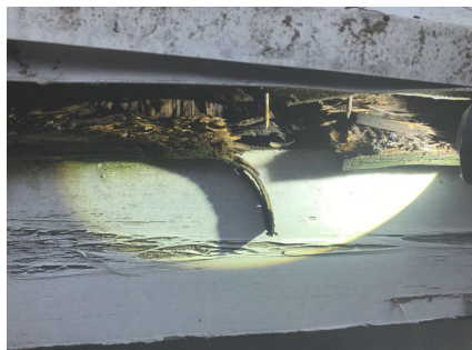
Deteriorated Roof Sheathing
