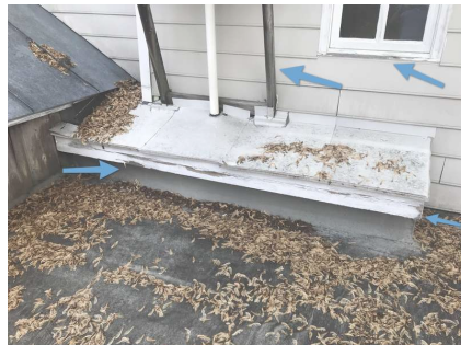
Wood Trim Needs Paint
