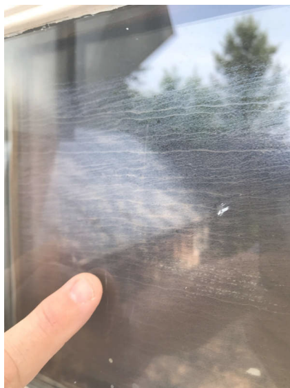
Failed Seal Close View
