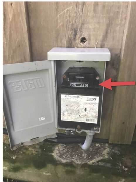
Heat Pump Emergency Disconnect
