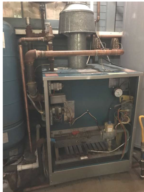
Front Cover Removed For Inspection
