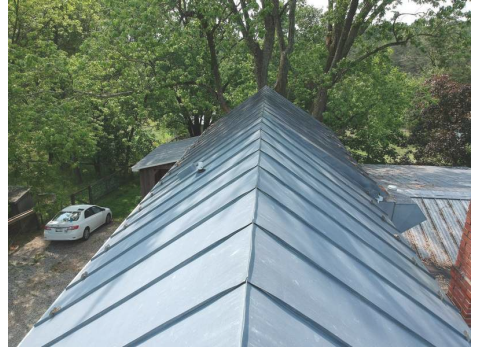
Metal Roof Ridge
