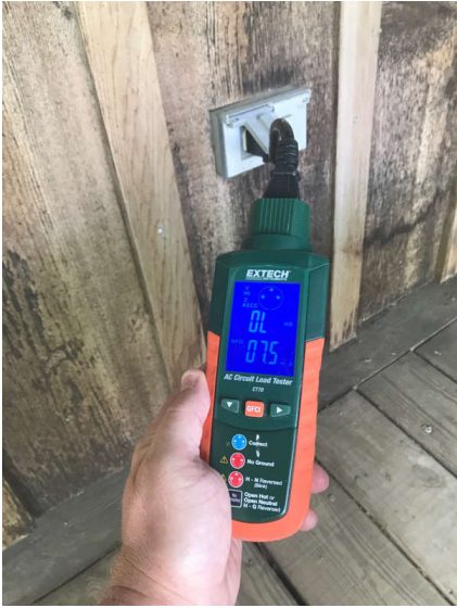
No GFCI On Front Porch
