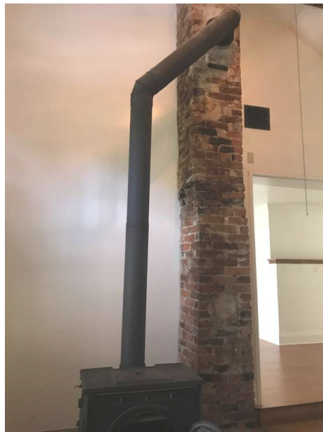
Wood Burning Stove Flue
