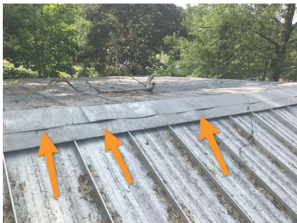
Unsealed Areas Of Ridge Vent
