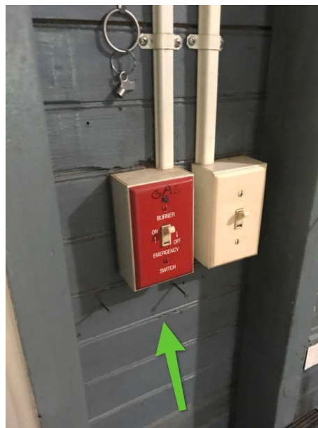
Boiler Shut Off Switch
