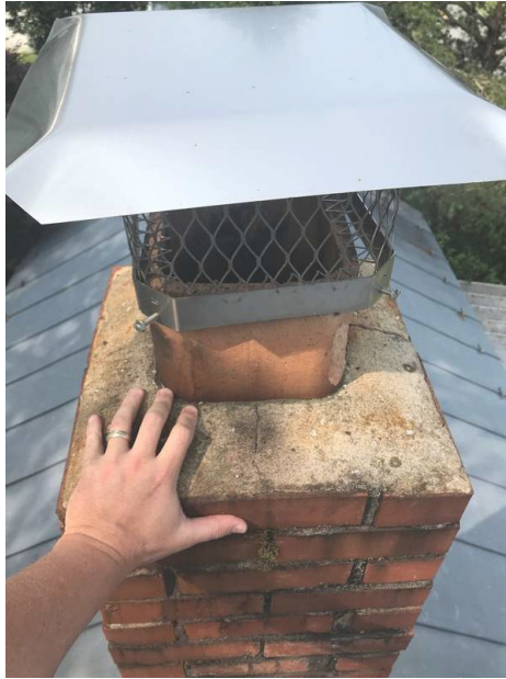
Chimney Crown / Cap
