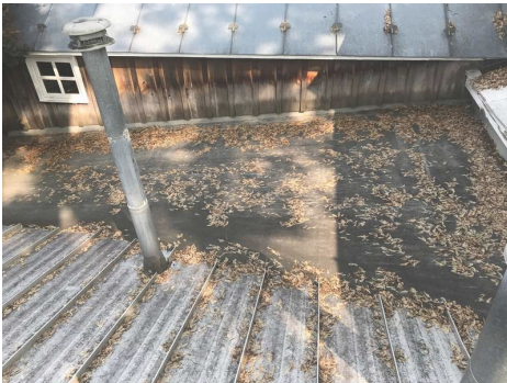
Rubber Membrane Roof Covered Area
