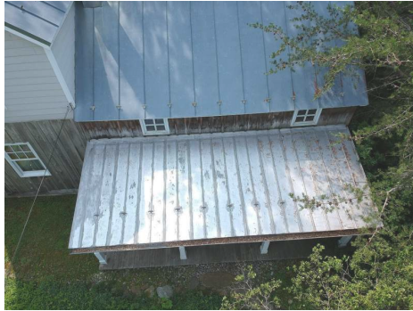
Front Aerial View
