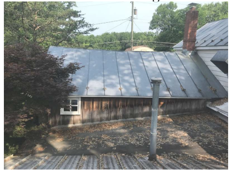
Rubber Membrane Covered Roof Area
