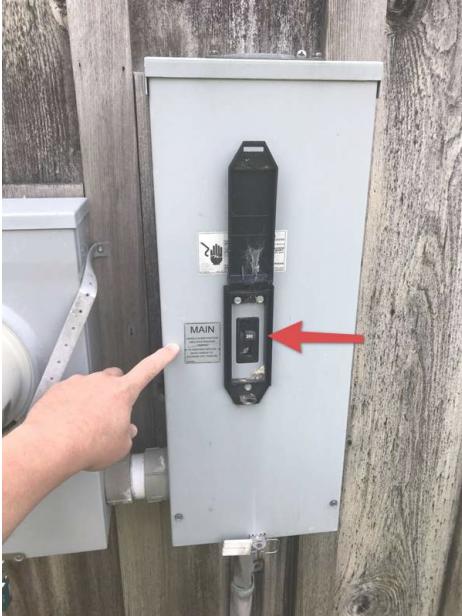
Main Electrical Disconnect (Exterior Front)
