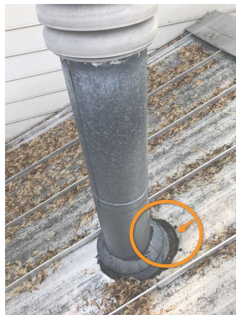
Roof Sealant Traps Water
