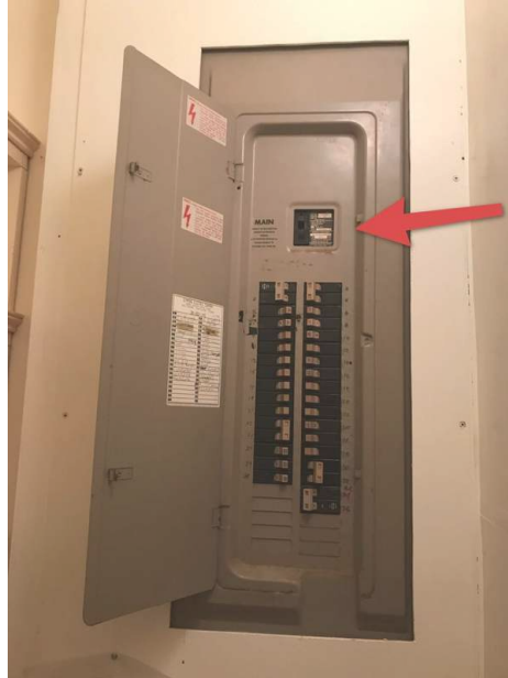
Main Electrical Disconnect Inside Electrical Panel
