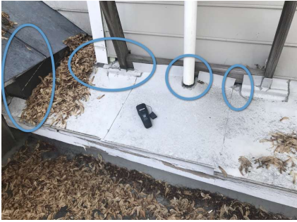
Improper Flashing
