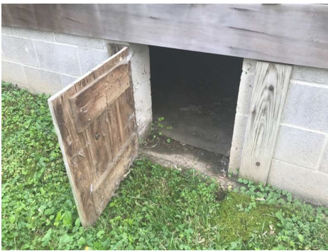
Exterior Crawlspace Access
