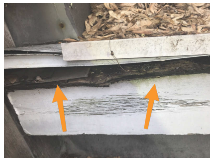
Deteriorated Roof Sheathing
