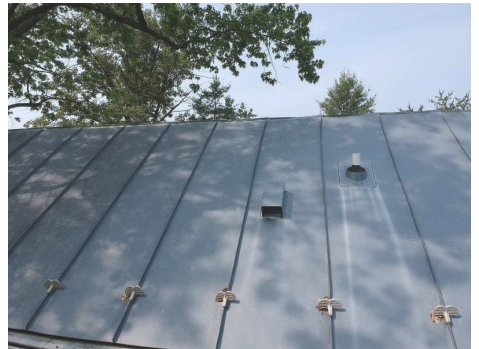
Metal Roof Plumbing And Bath Fan Vents
