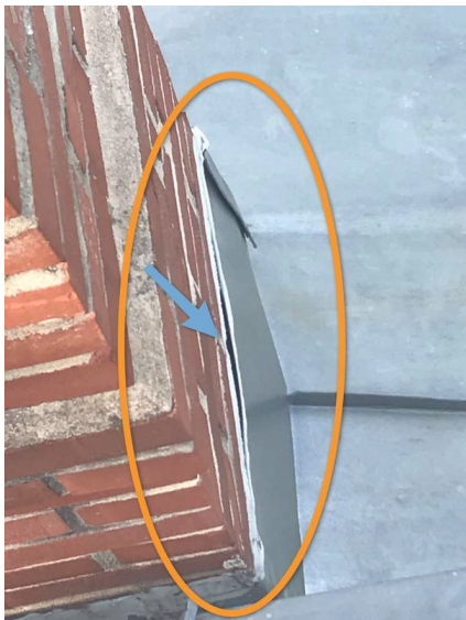
Chimney Flashing Separated From Masonry
