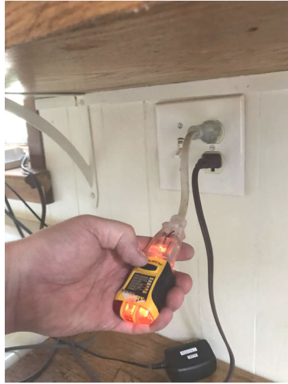
No GFCI In Kitchen (Near Sink)
