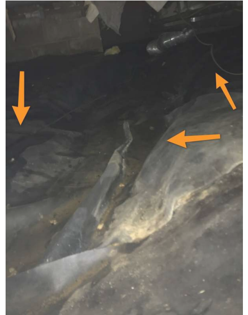
Standing Water In Crawlspace
