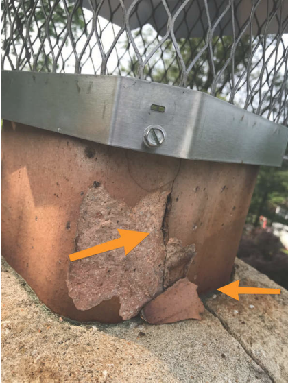
Cracked Chimney Flue
