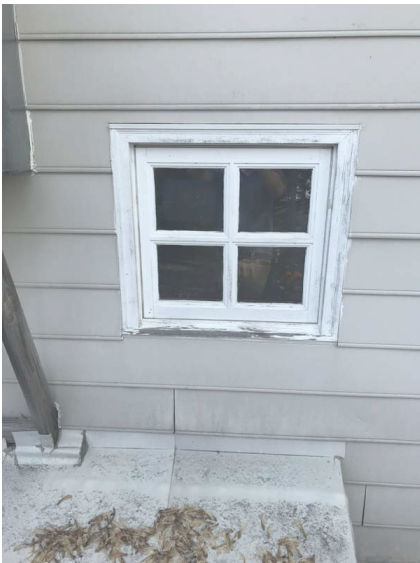
Wood Trim Needs Paint
