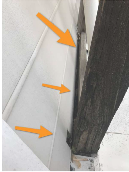
Missing Flashing / Unsealed Penetrations
