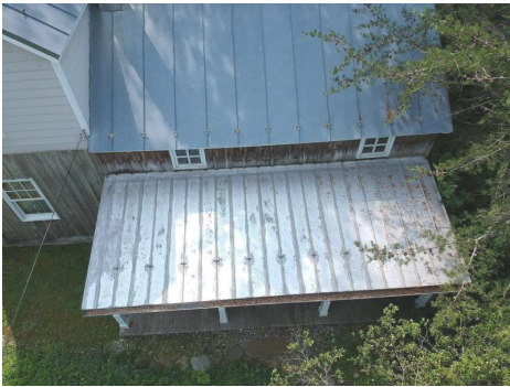
Front Porch Roof
