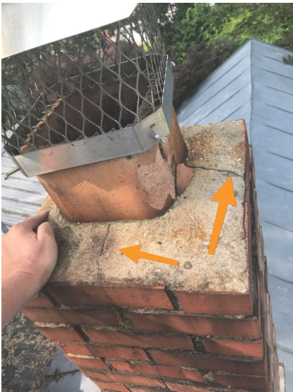
Cracked Chimney Crown
