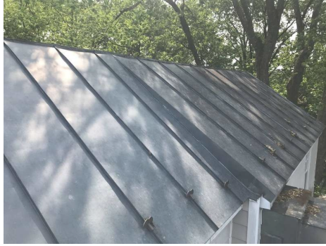
Metal Roof View
