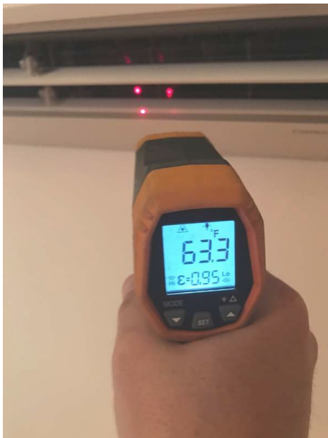
Conditioned Air Measured At 63 Degrees
