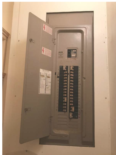
Main Electrical Panel, 200 Amp Service
