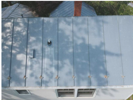
Roof Drone View
