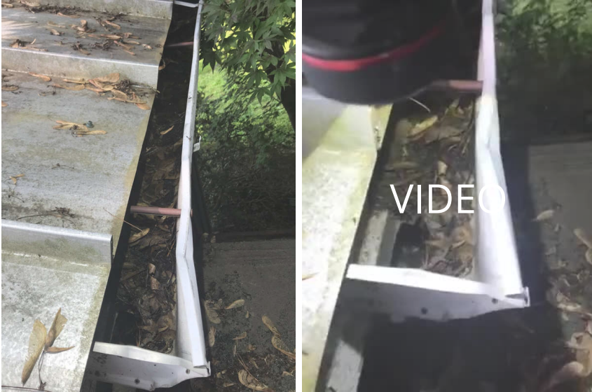
Debris In Gutters
