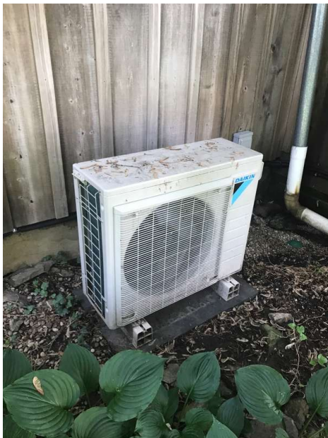
Heat Pump Condensing Unit
