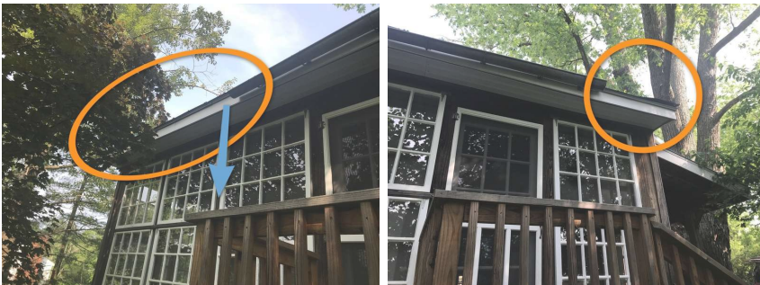
Missing Gutter And Downspout
