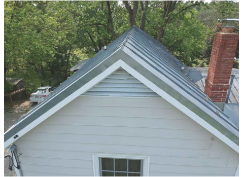
Front Aerial View
