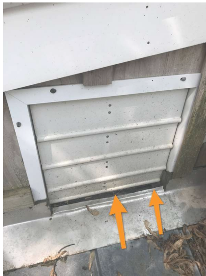
Gap In Flashing Below Sunroom Vent Fan
