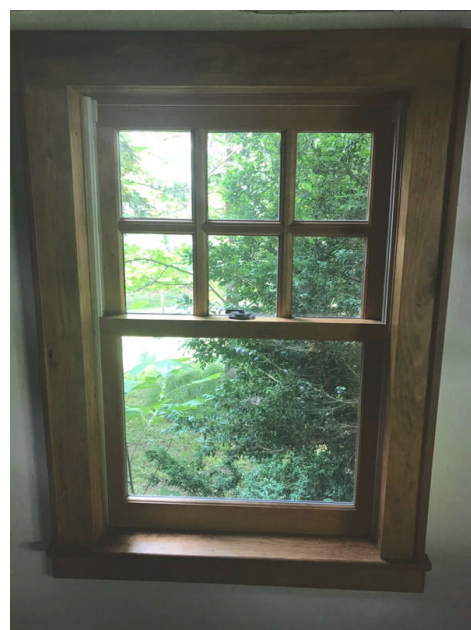
Window Screen Missing
