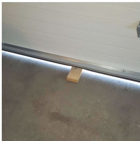
Safety reverse not operating
