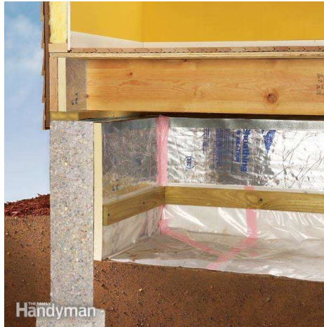
Extended up walls and sealed seams - ideal
