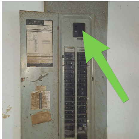
Main electrical shut off/disconnect
