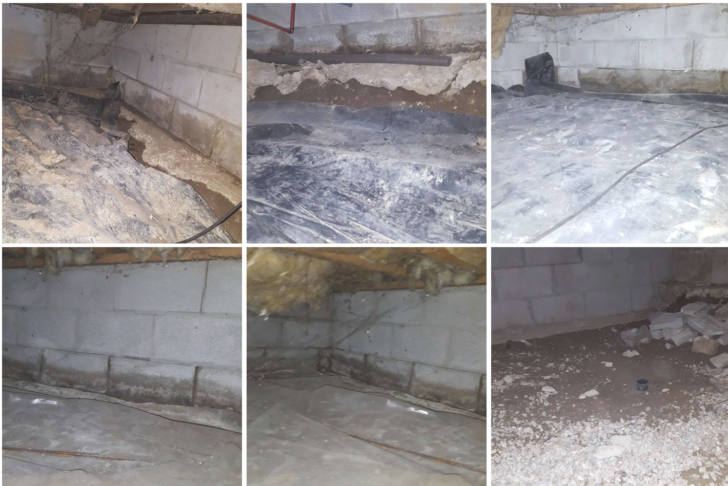
Addition - master bath area
