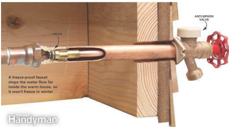
Frost free with anti-siphon
