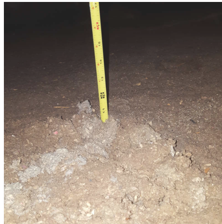
Insulation depth measurement
