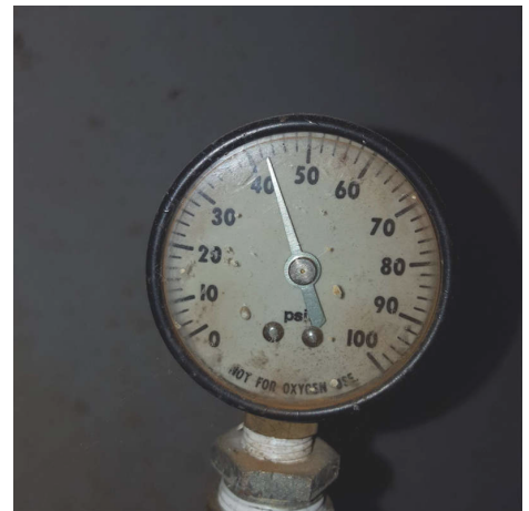
Static water pressure
