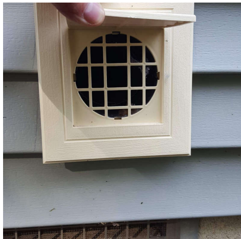
Easy fix - cut out plastic screen
