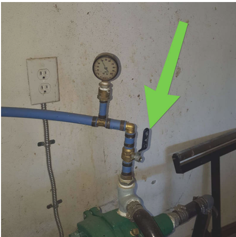
Main water shut off valve
