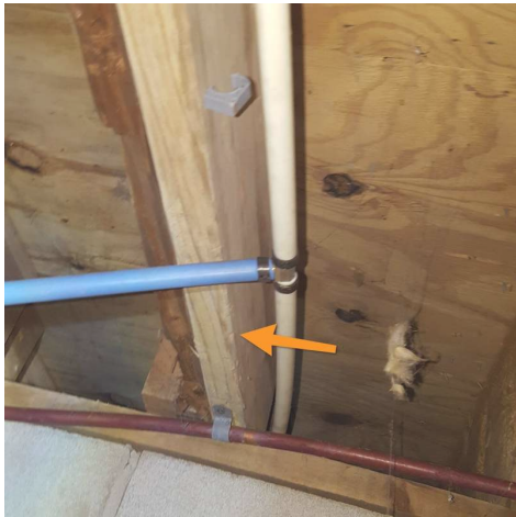
Newer "sistered" joist
