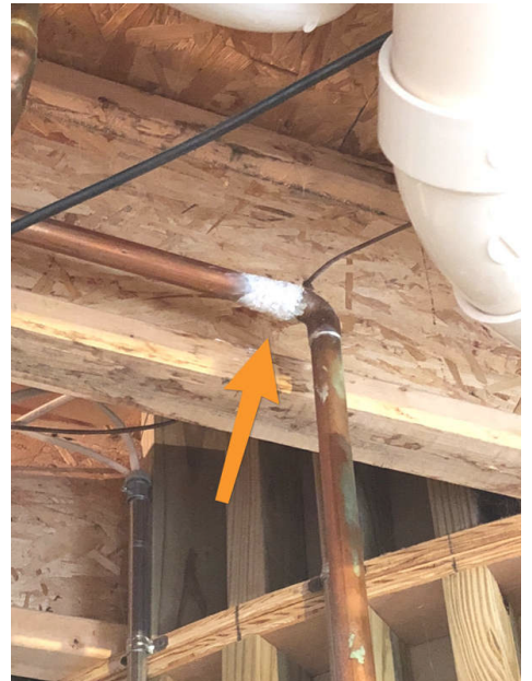
Above water heater. Basement
