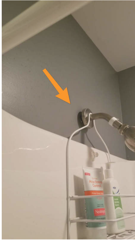
2nd Floor Bathroom
