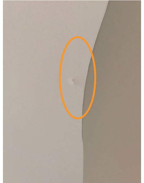
Behind stair well main ceiling
