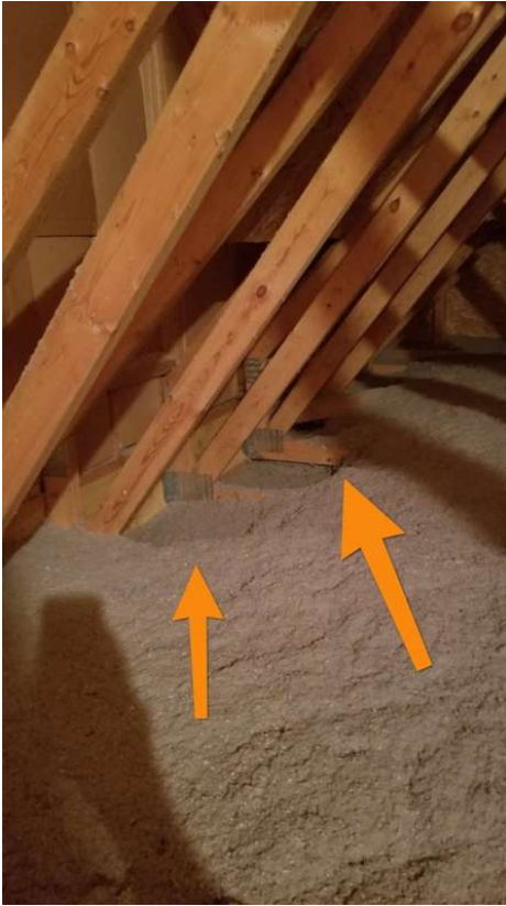
Attic Insulation: Insulation Type Blown
