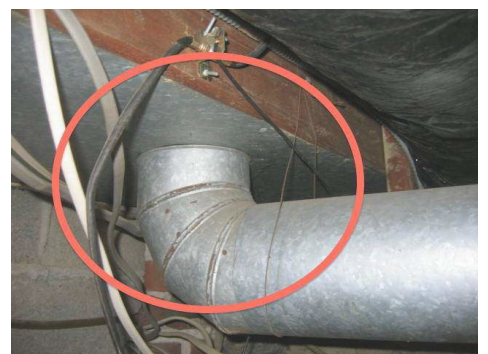
Loose connection; recommend sealing.
