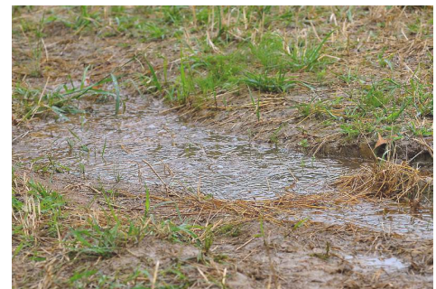
Water pooling in yard; recommend drainage
