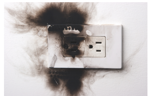
Scorch marks on cover plate
