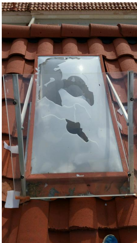
Broken skylight presents risk of water entry and glass shards entering house.
