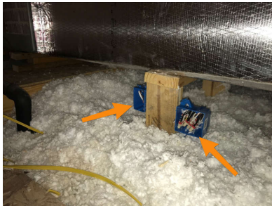
Attic Under AC Cabinet Plenum
