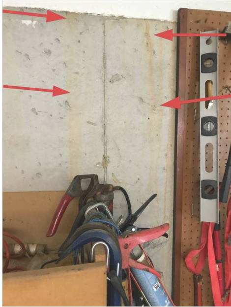
Moisture stains along the east foundation wall of the garage.
