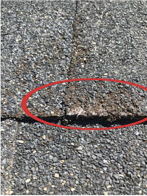
Damaged shingles.
