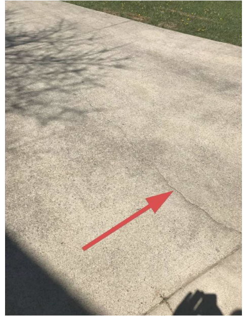
Minor driveway crack.
