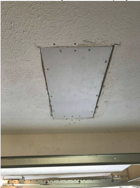
Area in garage needs to be properly patched.
