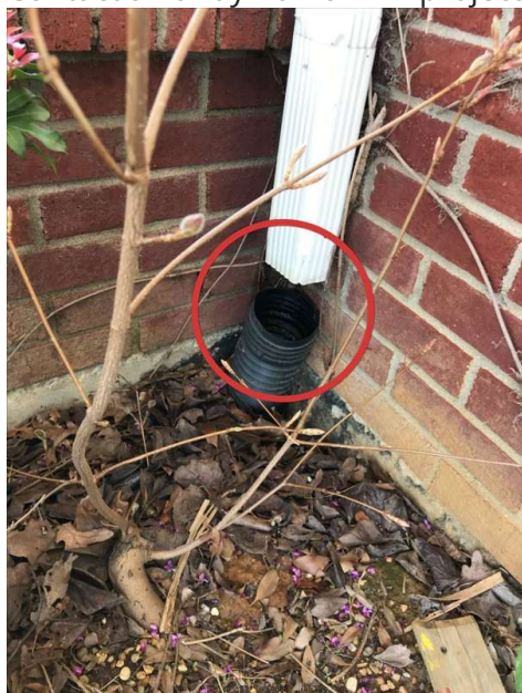
Recommend extending the downspout into the drain pipe.
