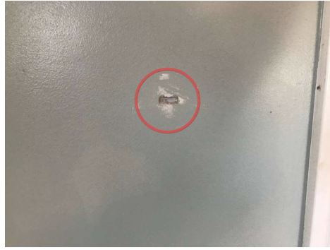
Doorknob hole, kitchen basement door.
