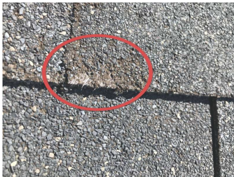
Damaged shingles.
