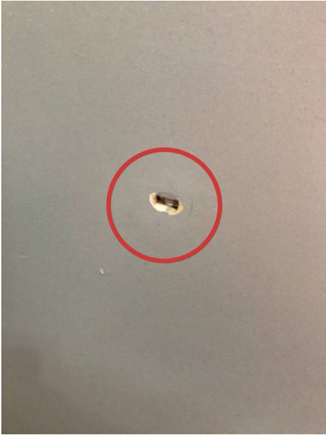
Doorknob hole, living room front door.
