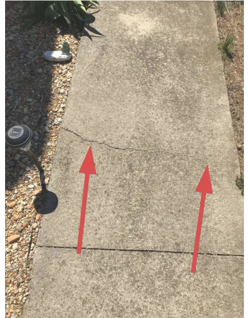
Minor walkway crack.
