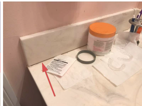
Upstairs bathroom, caulk needed to prevent water intrusion.
