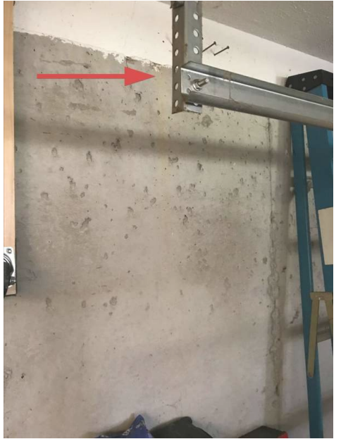
Moisture stains along the east foundation wall of the garage.
