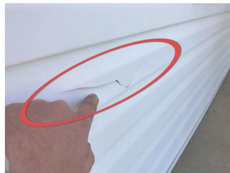
Minor crack is vinyl siding on front porch. Recommend repair or replace to prevent moisture intrusion.
