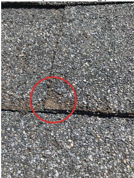
Damaged shingles.
