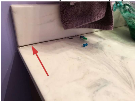
Master bathroom, caulk needed to prevent water intrusion.
