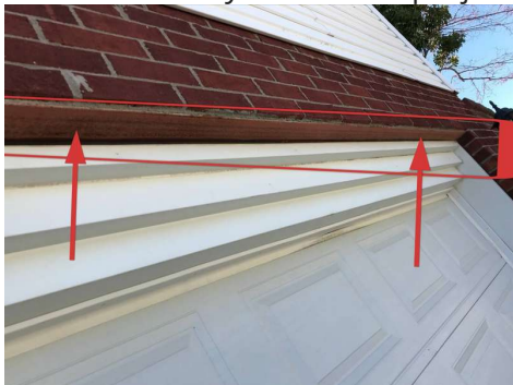
Metal lintel needs to be painted to prevent rust.
