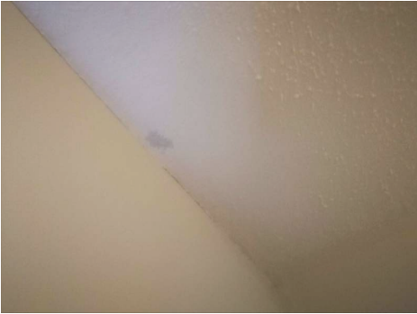
Poor Paint finishing observed
