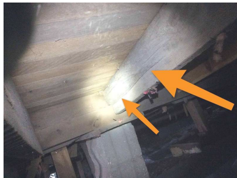
Joist have cracked
