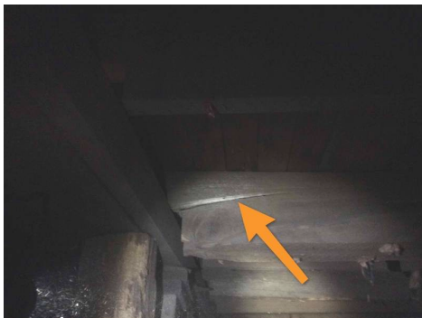
Joist has cracked
