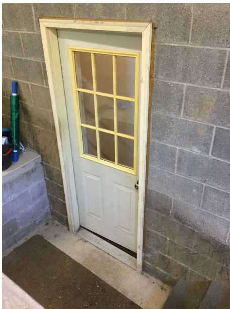
Occupant Door (From garage to inside of home): General
