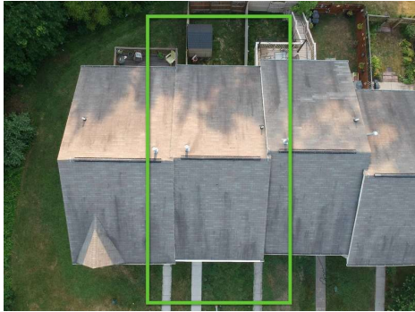
Aerial View of Roof
