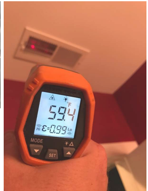
Conditioned Air Measured At 59 Degrees At First Floor Register
