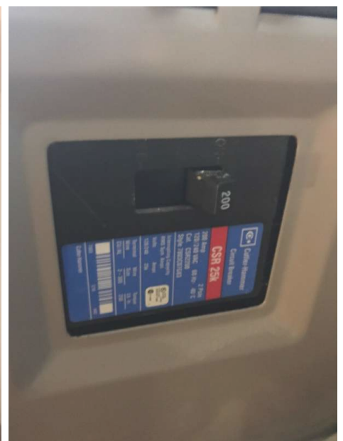
Main Electrical Shut Off Breaker
