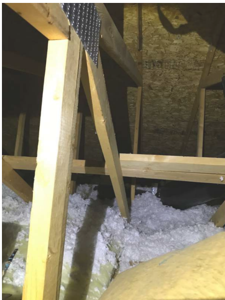
View of Attic Insulation and Roof Sheathing
