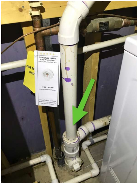
Main Sewer Drain
