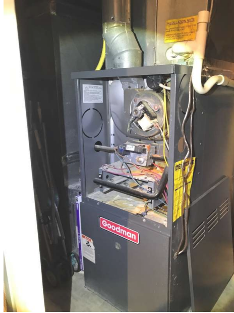
Gas Furnace With Cover Removed For Inspection
