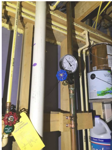
Fire Suppression System Pressure Gauge.
