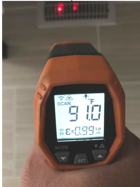
Heated Air From Furnace Measured at 91 Degrees at Kitchen Register
