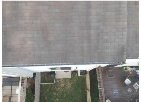
Rear Roof Coverings and Gutter
