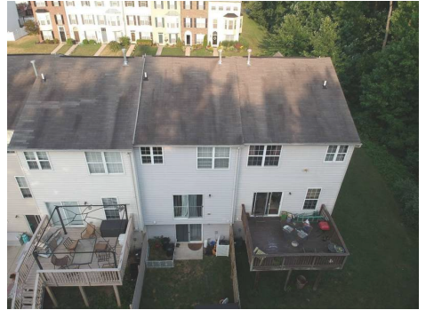
Rear Aerial View
