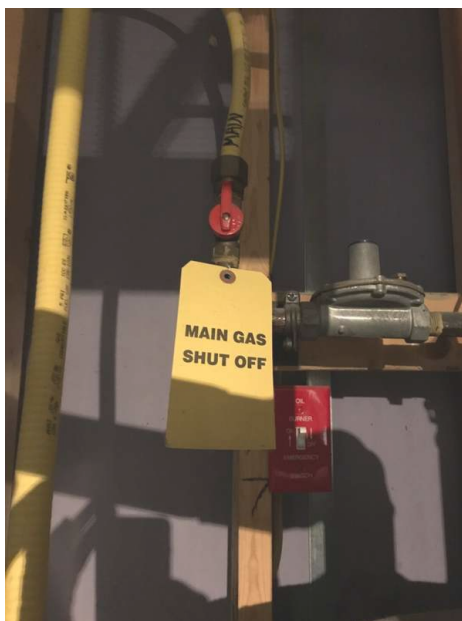
Main Gas Shut-Off Valve
