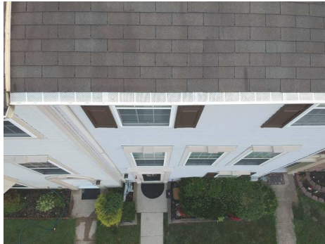
Front Gutter Protected By Gutter Guards
