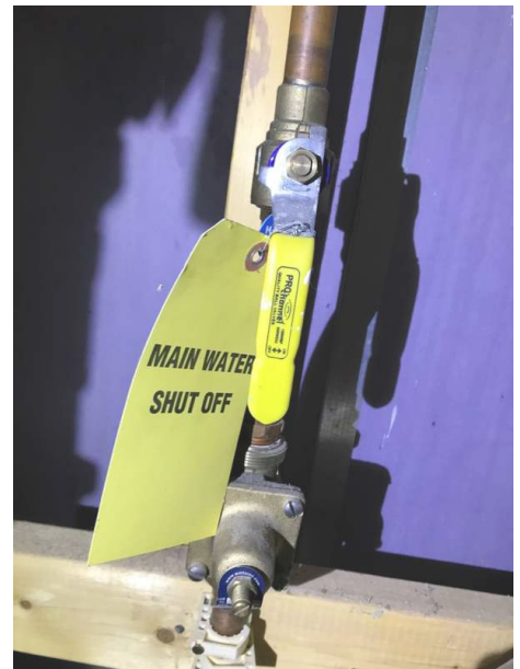
Main Water Shut Off Valve
