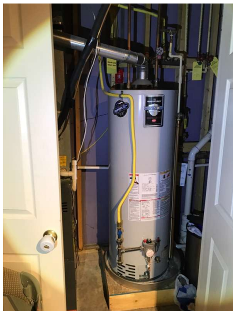
Gas Water Heater
