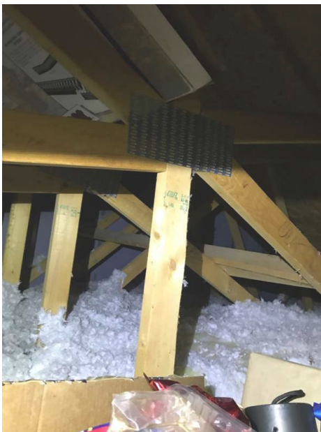
View of Attic Insulation and Roof Truss
