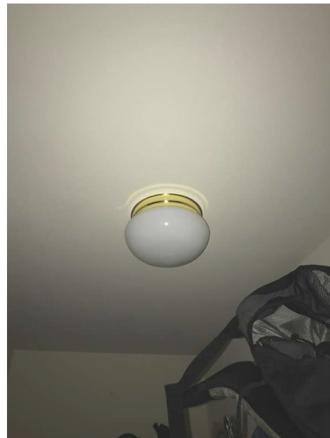
Inoperable Closet Light
