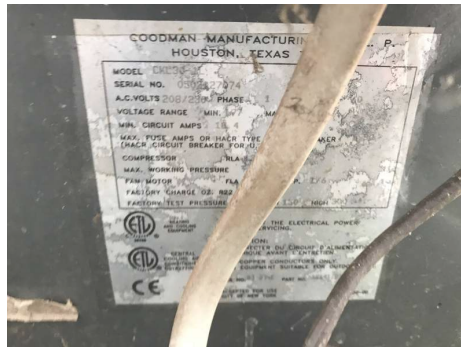
Air Conditioner Data Plate, Unit Manufactured in February 2005, 2.5 Ton Capacity
