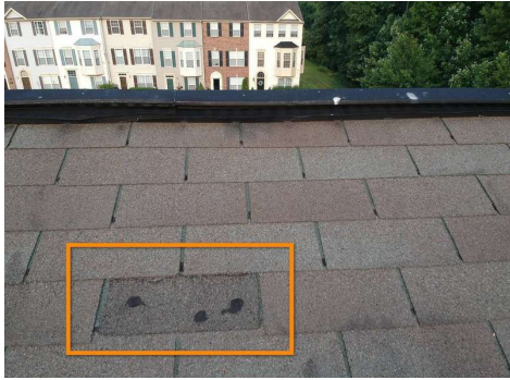
Missing Shingle (Rear Side of Roof)
