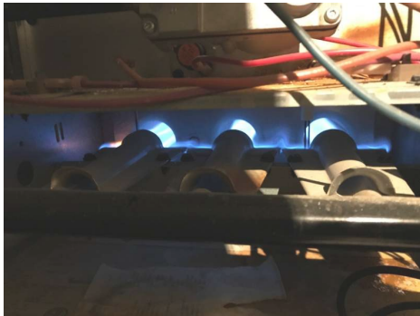
View of Gas Burners Operating In Furnace
