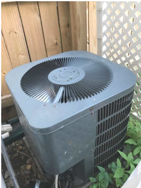
Air Conditioning Unit
