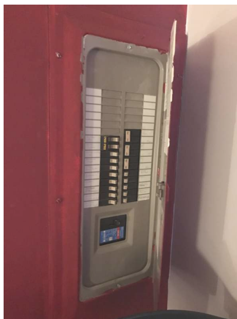
Main Electrical Panel Door Open
