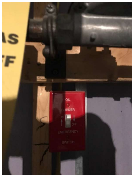
Furnace Emergency Shut-Off Switch
