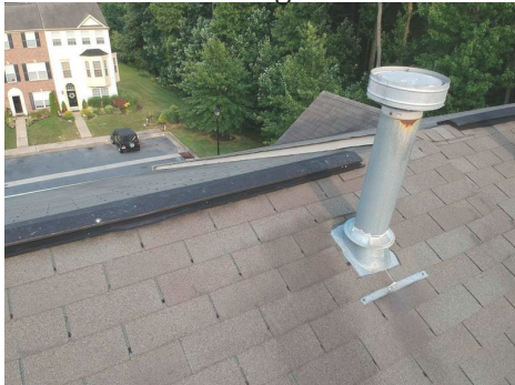
View of Chimney
