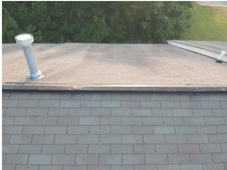
View of Ridge Vent, Chimney, and Plumbing Vent
