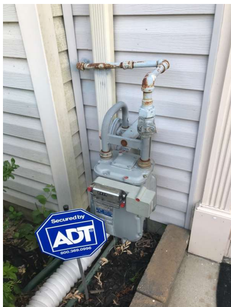
View of Gas Meter
