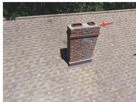
Chimney crown. Cracked mortar
