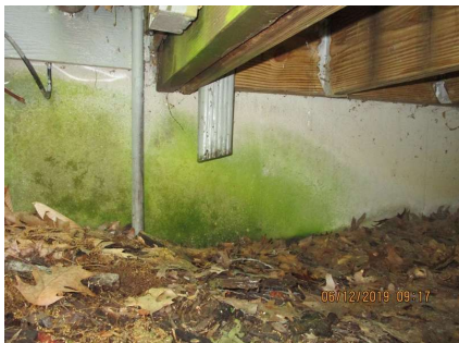
Downspout extension needed
