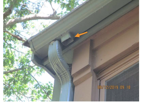
Gutter to downspout connection
