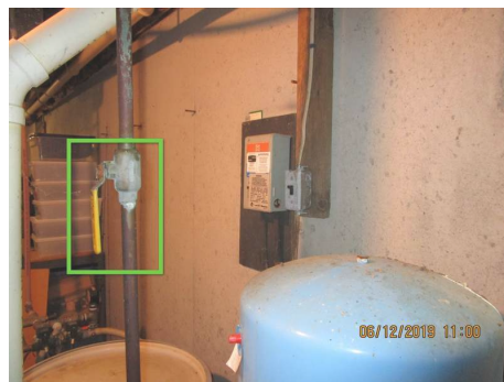
Main water shut-off valve
