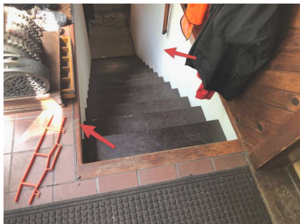
Missing railings and graspable handrails.
