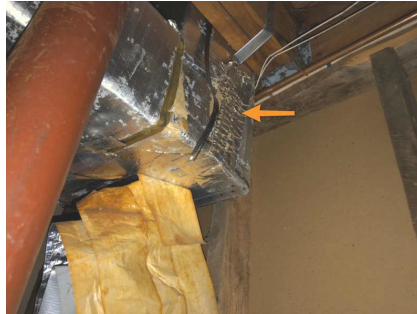
Insulation loose and falling off distribution ducts.
