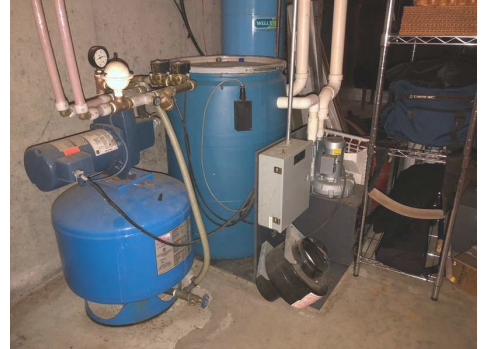
Radon water filtration system- AeroSparge 2000
