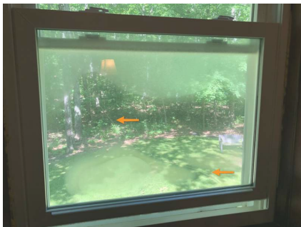
Crack in window. Failed seal
