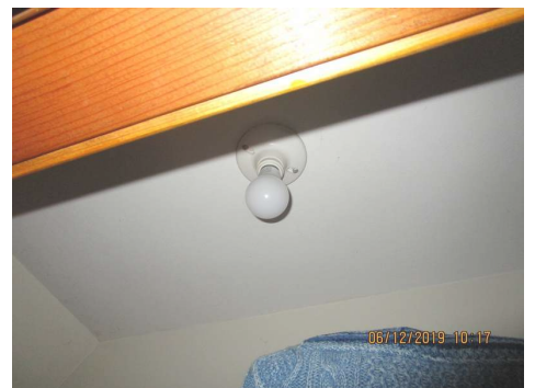
Improper and no switch located during inspection to activate fixture
