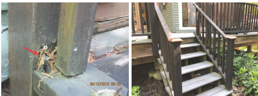
Railing damaged and loose.
