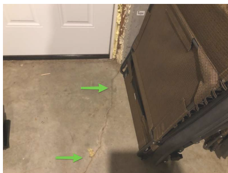
Shrinkage cracks
