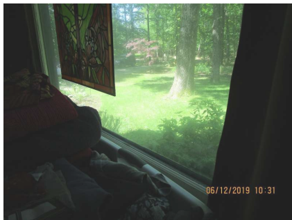
Failed Seal. Living Room
