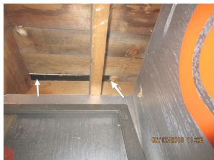
Sliding door. Basement view
