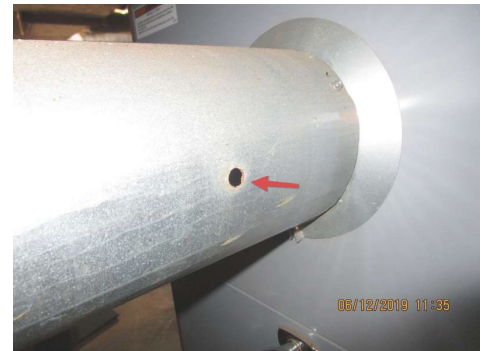
hole in flue vent pipe
