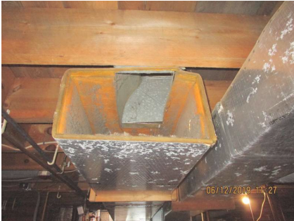
Missing end cap. Return air entering system from unconditioned basement
