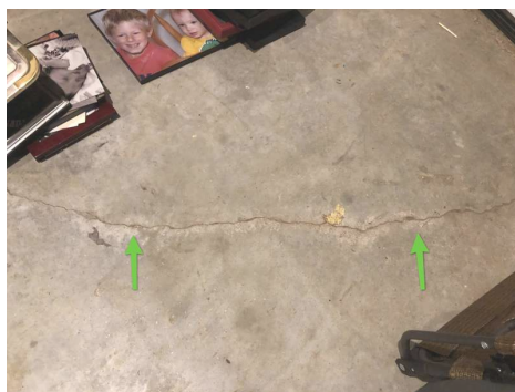
Cracks. Shrinkage
