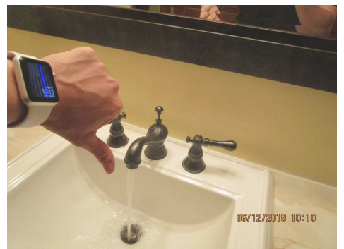
Drain stop inoperable
