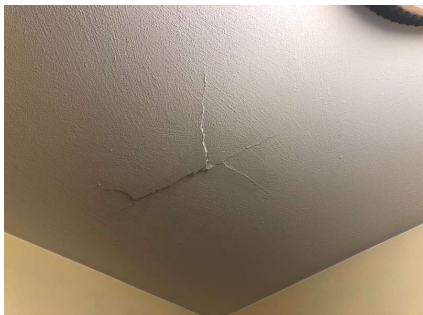
Crack in hallway. 2nd Floor
