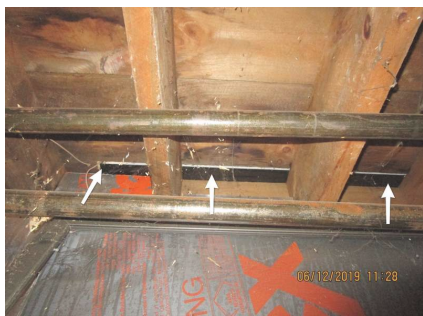
Sliding door. Basement view
