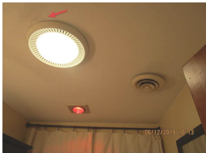
Stain observed in bathroom. 2nd Floor
