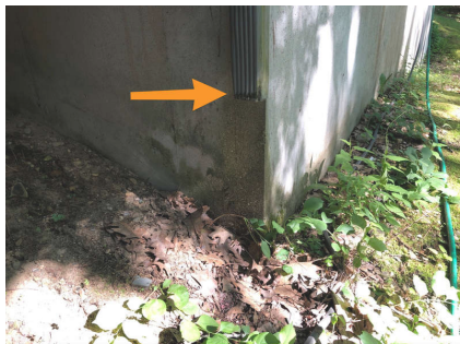
Downspout extension needed
