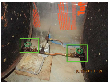
Main oil shut-off valves
