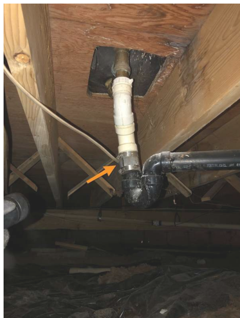
Correct way to connect ABS to PVC pipe
