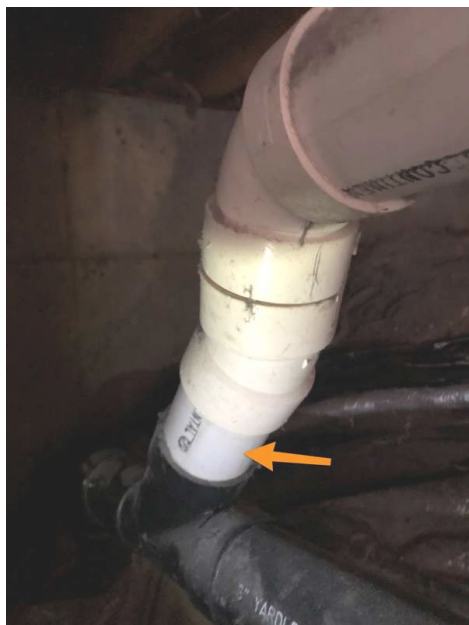
Incorrect way to connect PVC to ABS pipe. Can't be glued.
