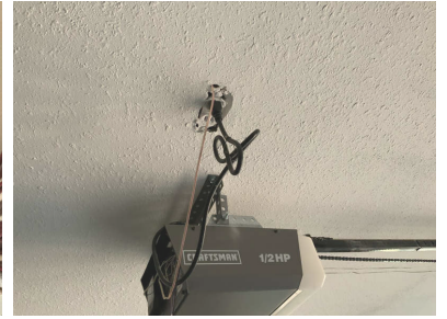
Garage door opener receptacle.
