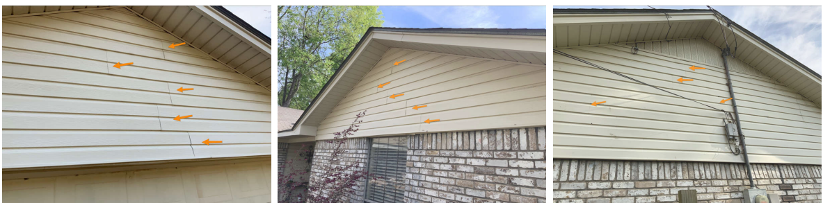
Over garage door
