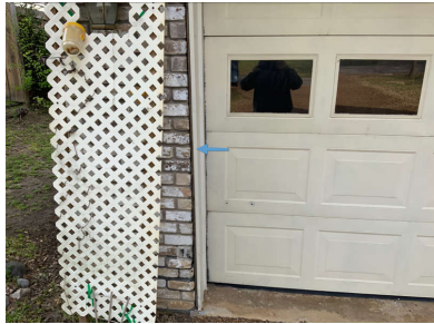
Left side of garage door trim
