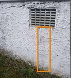
4.1.2 Perimeter wall - Concrete CRACKING - SUPERFICIAL The solid plaster coating in some isolated areas are showing some cracks, these are drumming when tapped. This is superficial, not structural cracking. if left, should not cause any future problems to the foundation itself.
