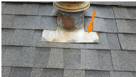
Loose, nail heads exposed
