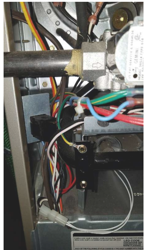
Wrong place for safety switch.
