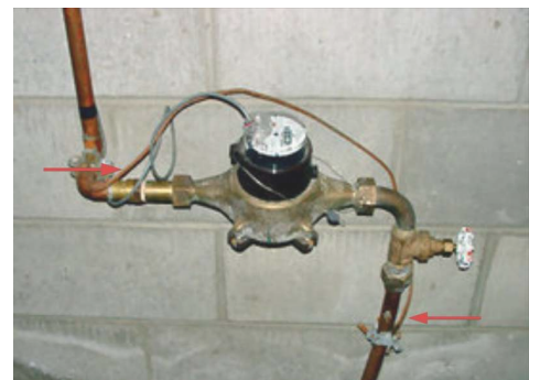
Example of a bonding jumper at the water meter
