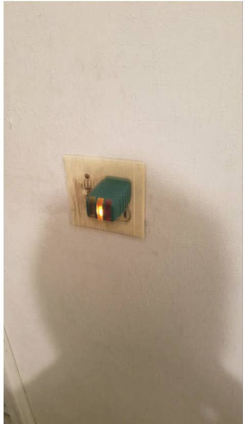
Garage, right of house door
