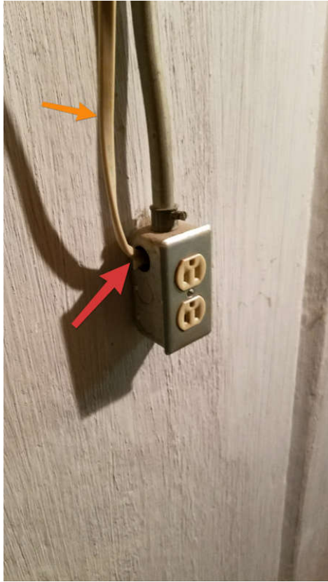
Also note missing cable clamp
