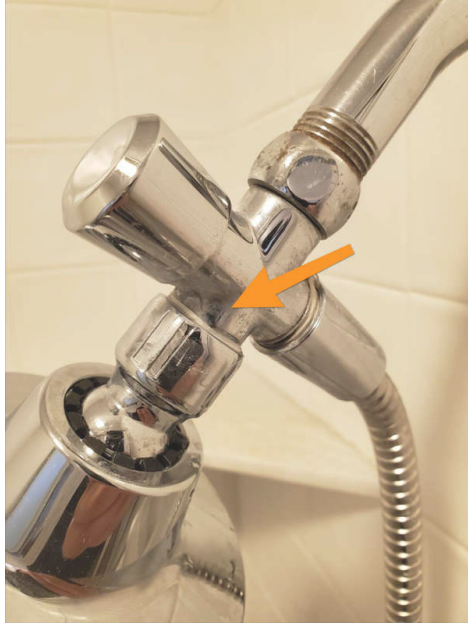
Leak at fitting - master
