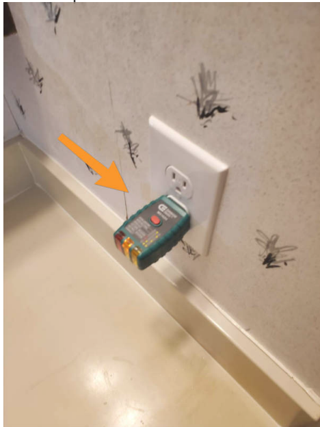
Right Side master sink
