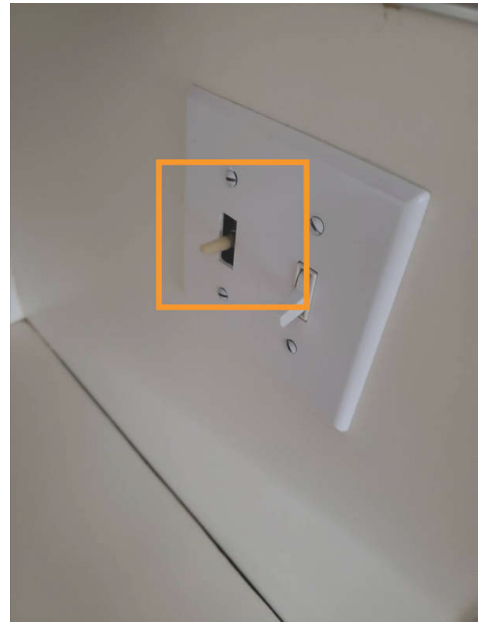
Control kitchen ceiling fan speed
