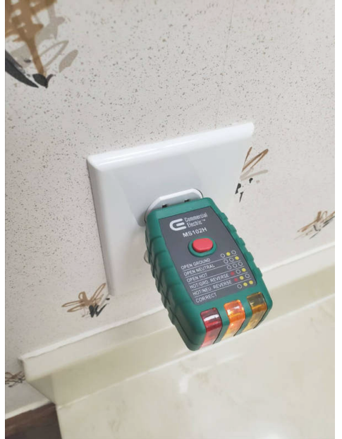
Hallway bathroom - left of sink
