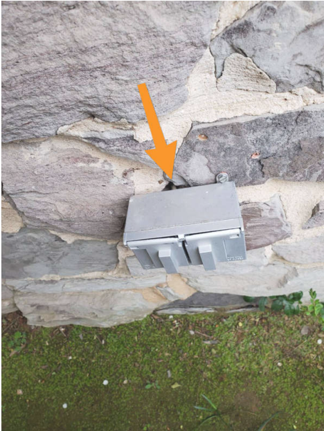
Front right side - loose and needs secured
