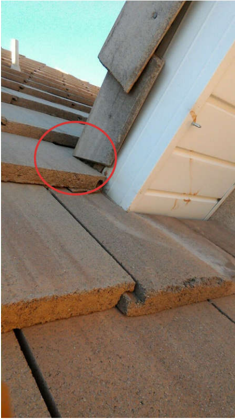
Near corner of garage and front room. There is no diverter.
