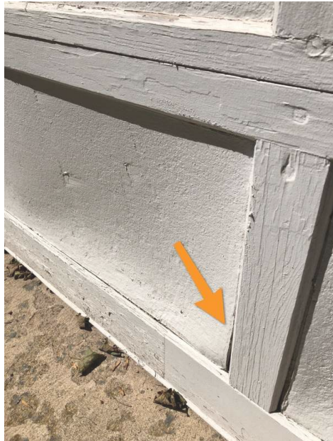
The shadow line should be straight, in this photo the line is highlighting the condition of the door by the visible waviness.
