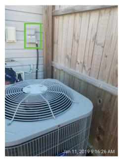
**Cooling Equipment and Operation: Cooling capacity** 24000 BTU/hr, 2 Tons
