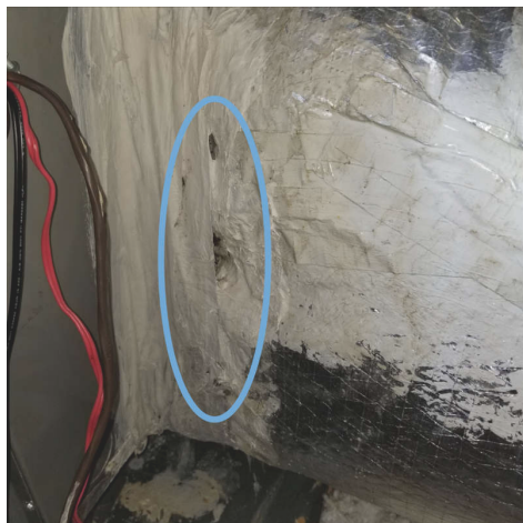
Right side of air Handler
