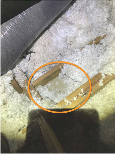
Above Laundry Room Hallway
