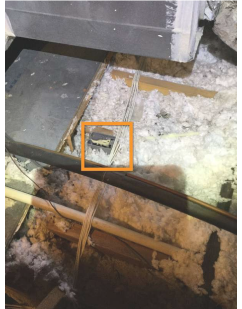
Front right of furnace
