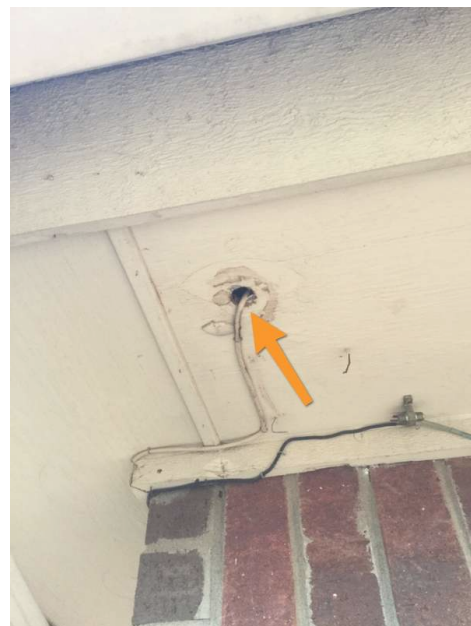
Northwest Corner Soffit
