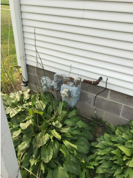
Main Gas Shut Off Gas Meter Outside
