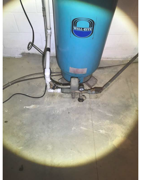
Main Water Shut Off Valve Basement, At The Well Pump
