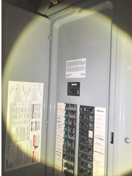
Main Electrical Shut Off At The Main Panel, Basement
