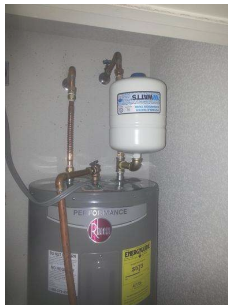
Example of an Expansion Tank at Water Heater
