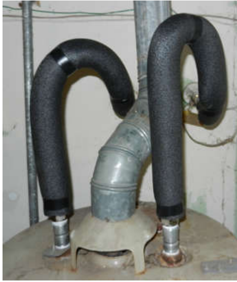
Example of Pipe Insulation at Water Supply Pipes
