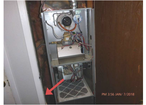
Make up air vents on left side of furnace. Direct line to garage.
