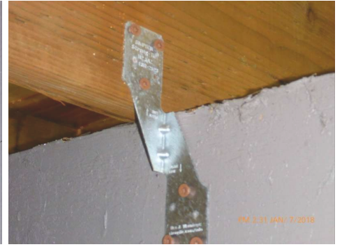
Beam-to-joist
