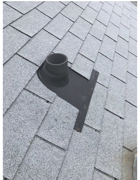
North facing roof on south side of house
