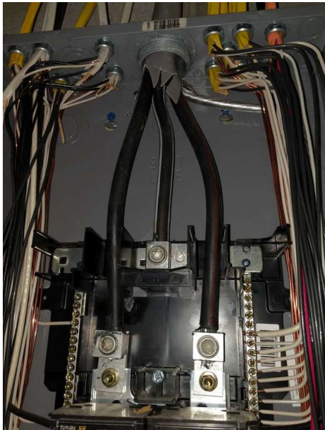
Main & Subpanels, Service & Grounding, Main Overcurrent Device: Panel Type Circuit Breaker
