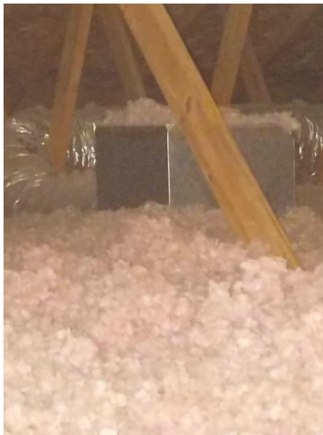
Distribution Systems: Ductwork - Distribution Insulated
