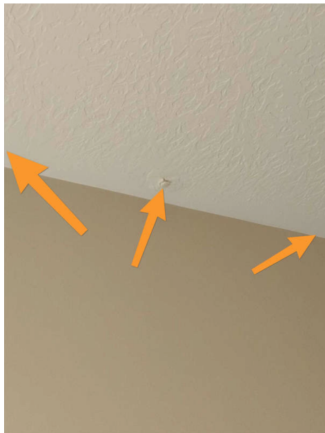
1st Floor Bathroom
