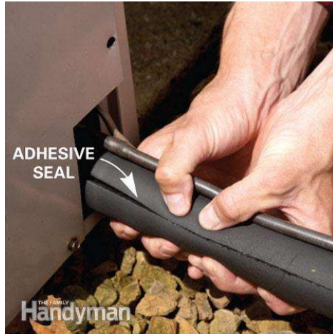
Add insulation to refrigerant lines
