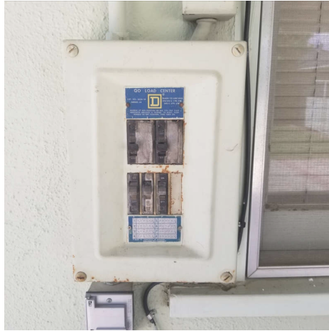
Exterior Sub Panel
