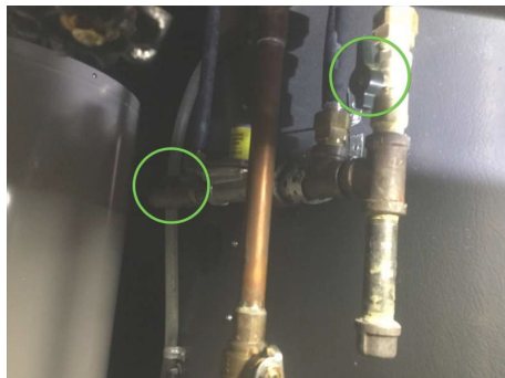
Gas Shut Off for furnace Right side off furnace
