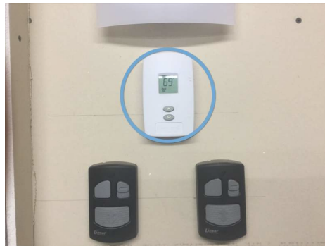
Thermostat for garage furnace
