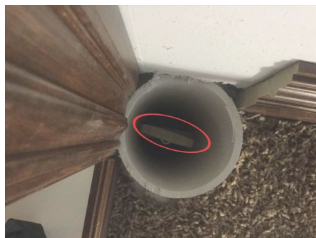
Gate Valve for closing off main sewer in case of Flood/Sewer Back-up
