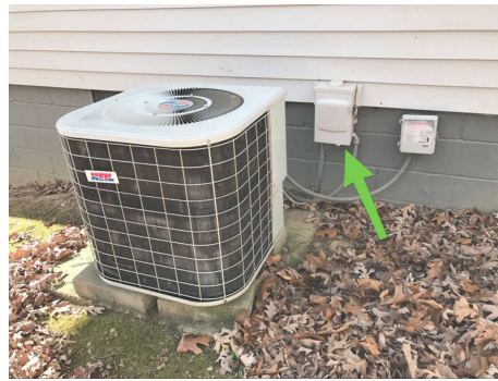
Condenser w/ cut off
