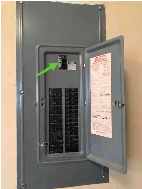
Garage Utility Room
