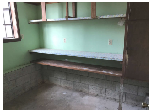
Garage Utility Room
