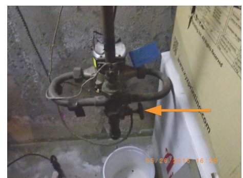
Main water shut-off location
