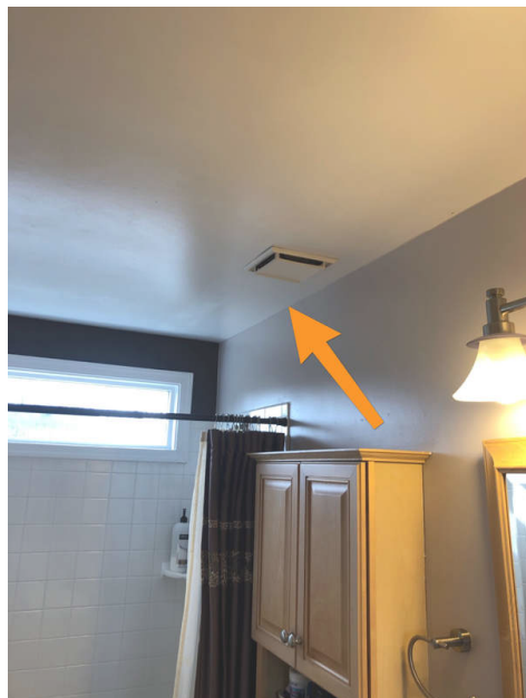
2nd floor Bathroom
