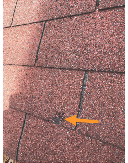
Rear garage near gutter edge
