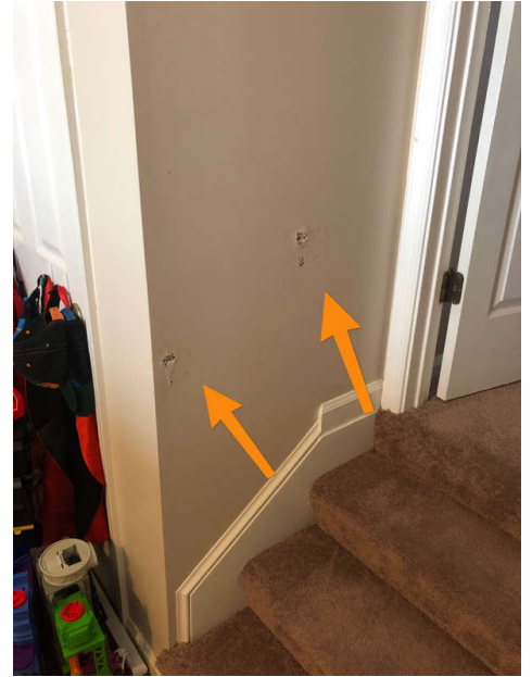
2nd floor above garage
