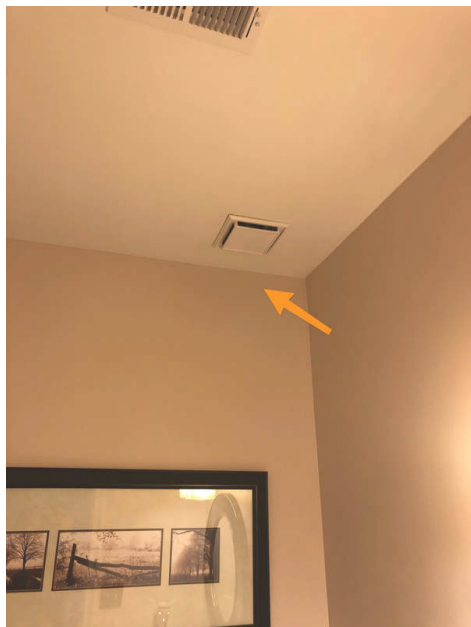
1st Floor Bathroom
