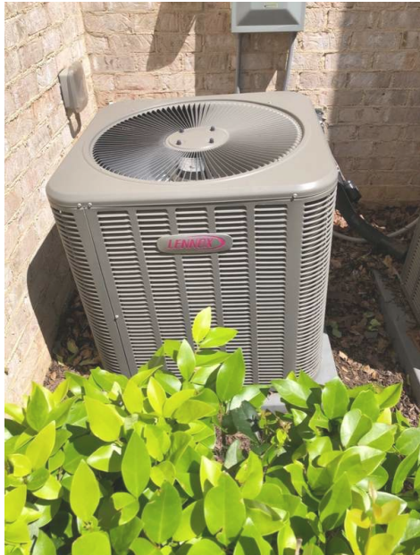
Bedroom Level Unit
