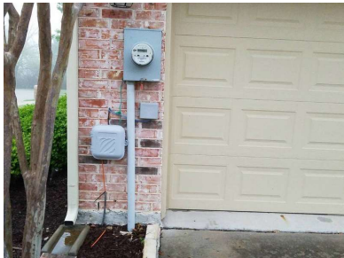
Type of Service Drop Wiring: Copper
