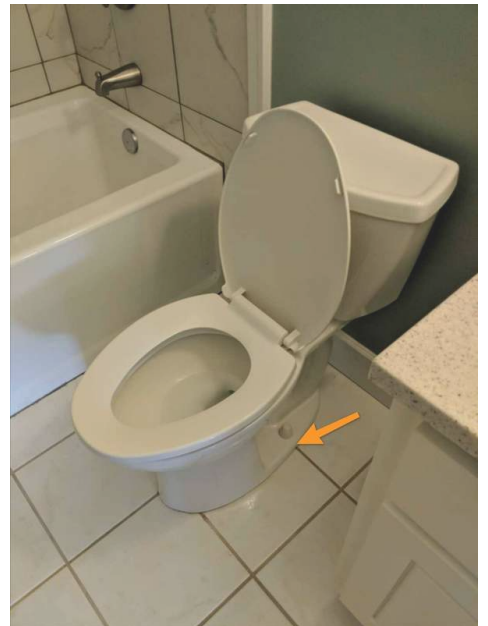
2nd Floor Bathroom
