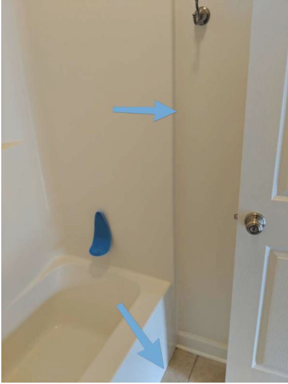
2nd Floor Bathroom
