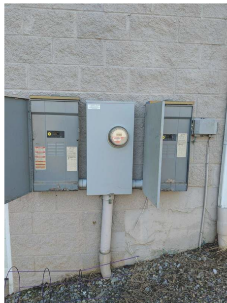
Main & Subpanels, Service & Grounding, Main Overcurrent Device: Main Electrical Disconnect Location At Service Meter, Exterior
