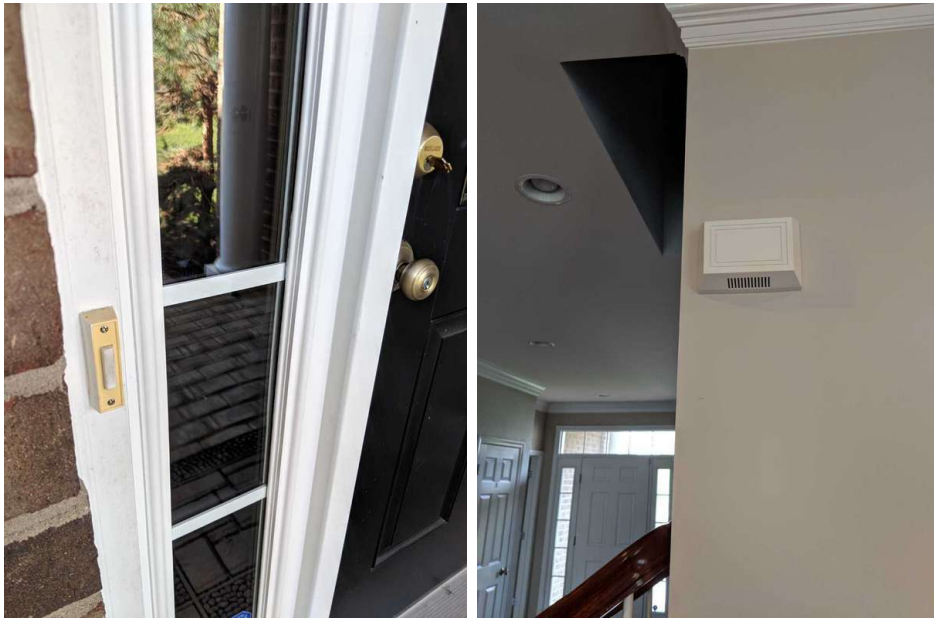
Lighting Fixtures, Switches & Receptacles: Lighting Fixtures and Ceiling Fans
