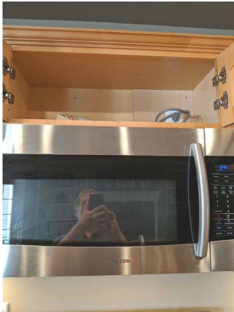
Range/Oven/Cooktop: Exhaust Hood Type Re-circulate, Over Range Microwave
