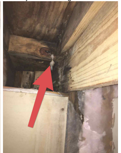
Floor joists showing deterioration
